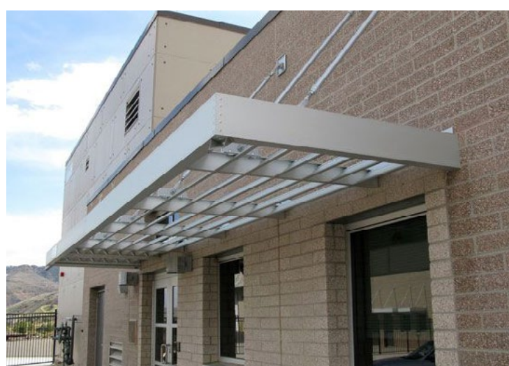
Modern awning structure, above all entrances
