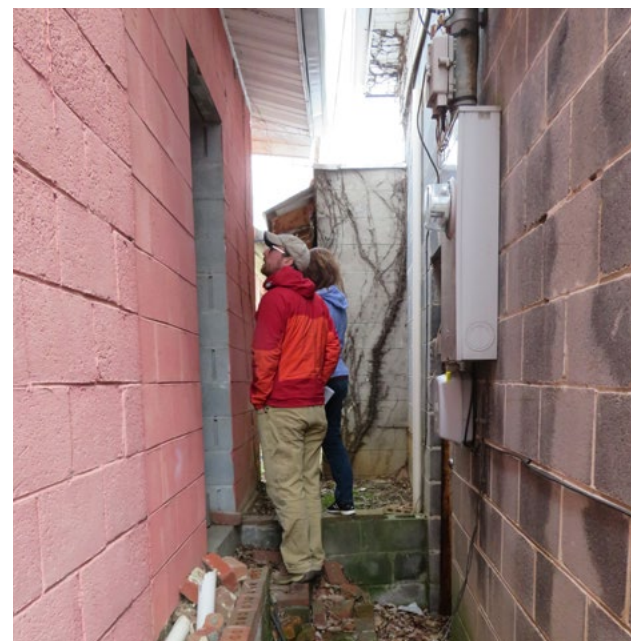
Narrow passage between the primary structure (right) and neighboring "pink building" (left).
