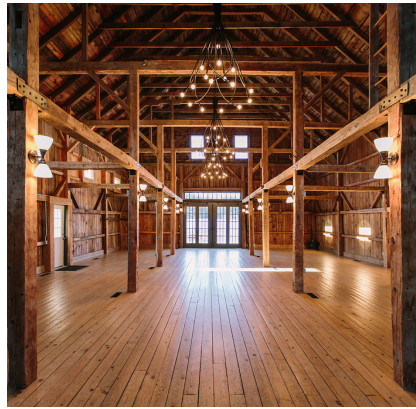
Interior Structural Support
