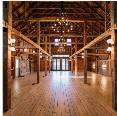
Interior Structural Support
