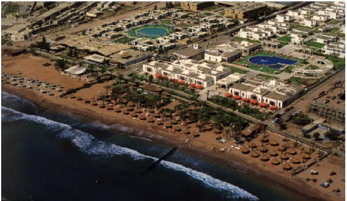
Fig.V.4. Hotel Construction on Beach in Naama Bay, Sharm El Sheikh Source: Isis Egypt, Sinai and the Red Sea:Pictoral Guide and Souvenir , Cairo 1996, p.25.
