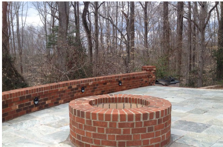
Brick Seating Wall
