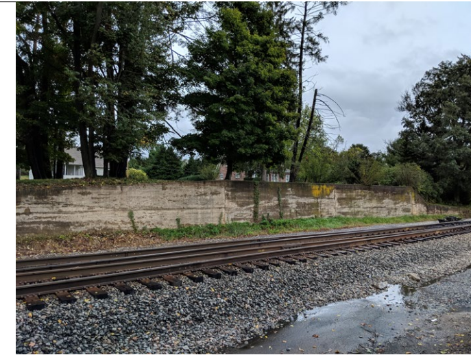
View of a concrete retaining wall adjacent to the railroad track, opposite of the trailhead site.
