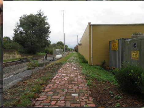
C. View of brick path behind senior center. This area should be designed with safety precautions put into place. The current brick path may not be easily accessible for people with disabilities or limited mobility, as well as bicycles. Wall of senior center is also well suited for a mural, making the site more visible. Safety fence should be added for the length of the trail.
