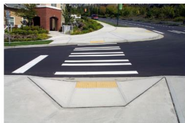
ADA Sidewalk & Pedestrian Crossing
