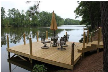
Creek Access + Steps + Deck
