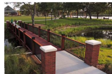
Pedestrian Bridge over Creek
