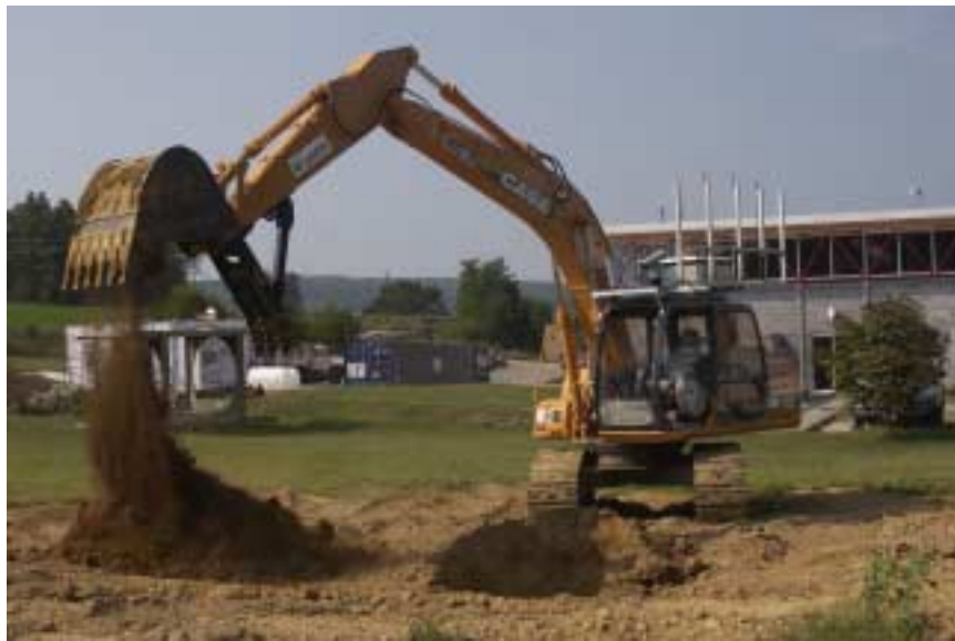
Figure 7.1: Teleoperated Case CX-160 excavator in operation
