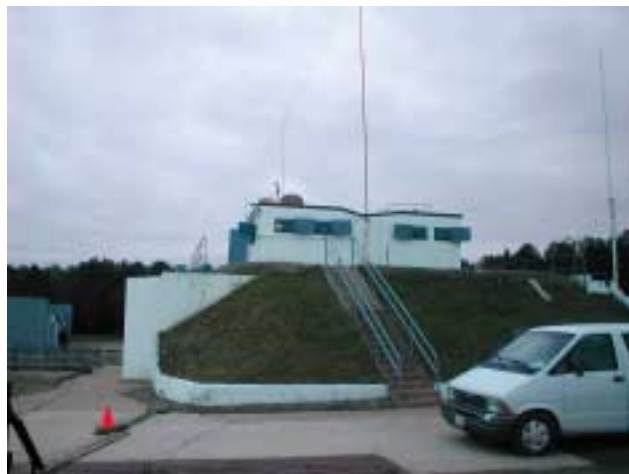
Figure 3.6: Remote station in Dahlgren, VA
