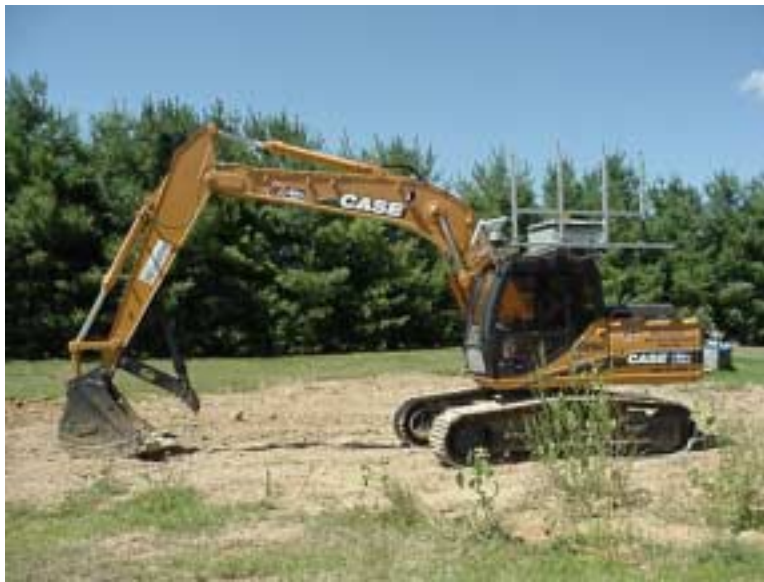
Figure 3.1: Teleoperated CX-160 excavator
