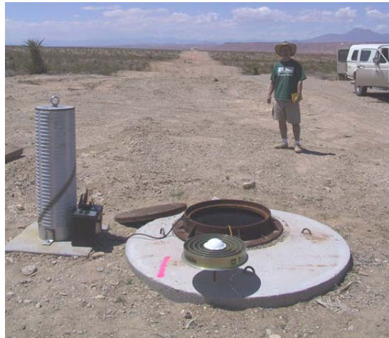
Figure 8: Antenna and receiver set up for stations VT1, VT3, VT4, VT6, VT10, and VT14 along the water line
