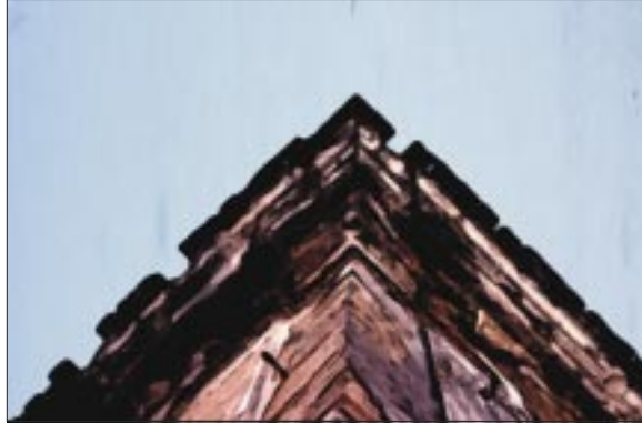
Cornice at corner of building
