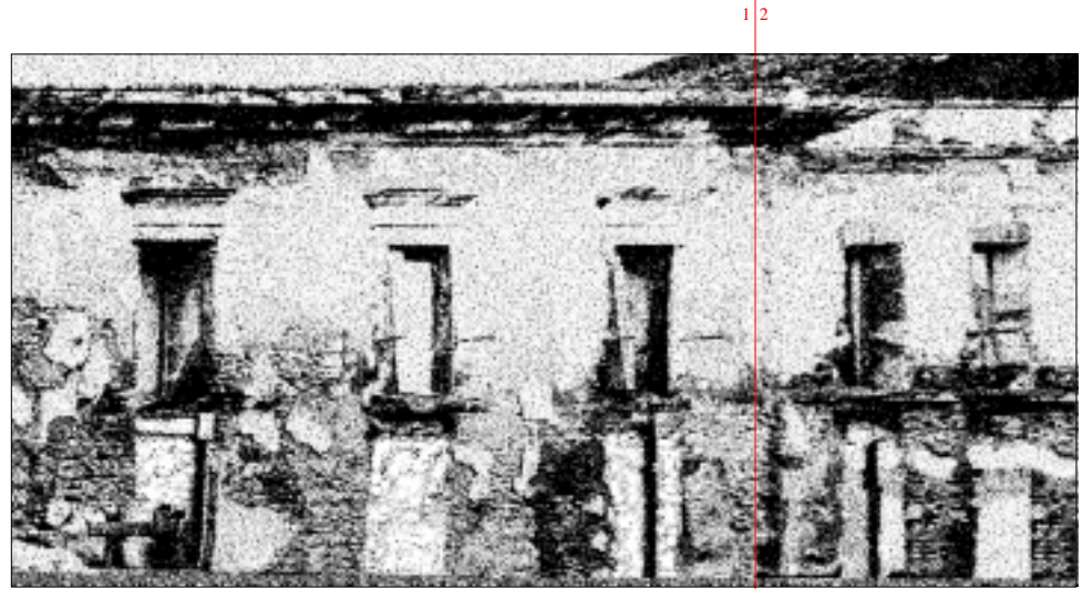
The north facade fronts San Sebastian street
