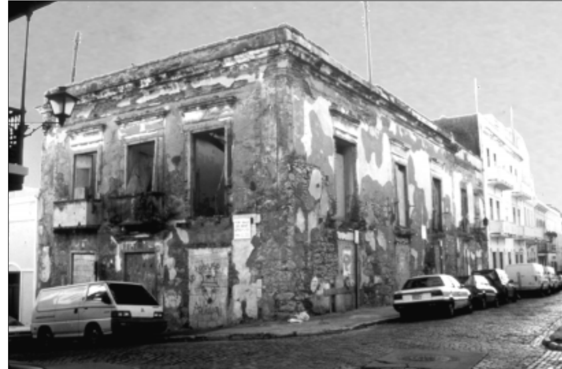
Northeast view of the existing building. Corner of San Sebastian st. and Cruz st.
