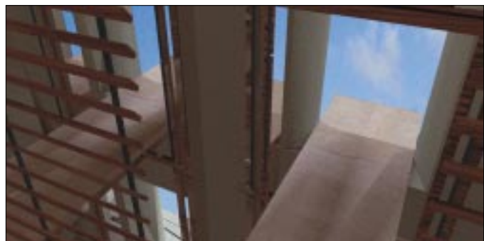
View from the third floor of the layered wall at the second floor balconies.
