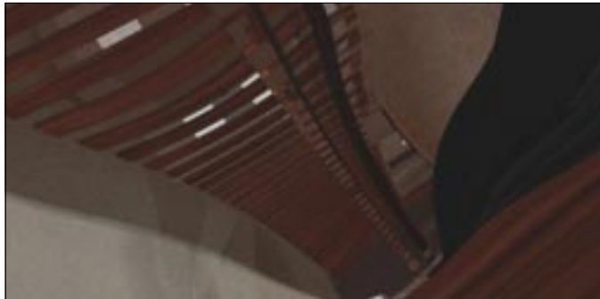
Looking down at the layered wall.
