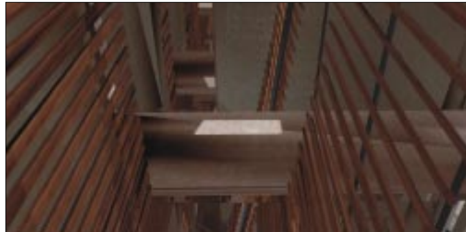
View from the layered wall at the bridges that intersects it.
