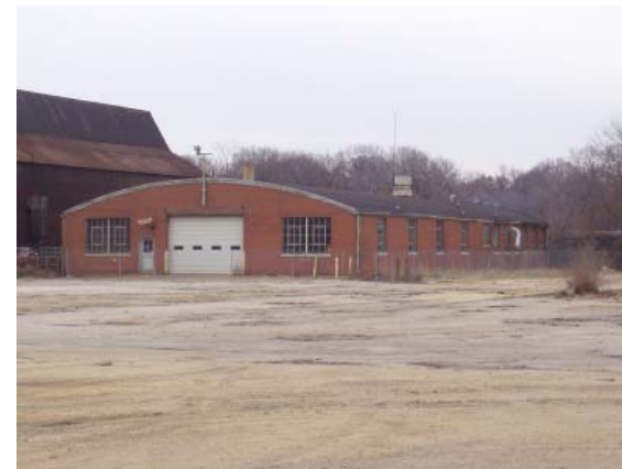
Figure 7.34. Front and side view facing west.
