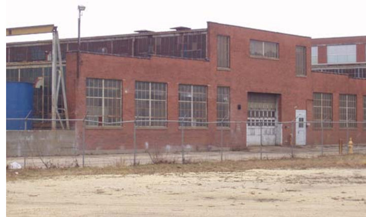
Figure 7.24. Building façade facing east.
