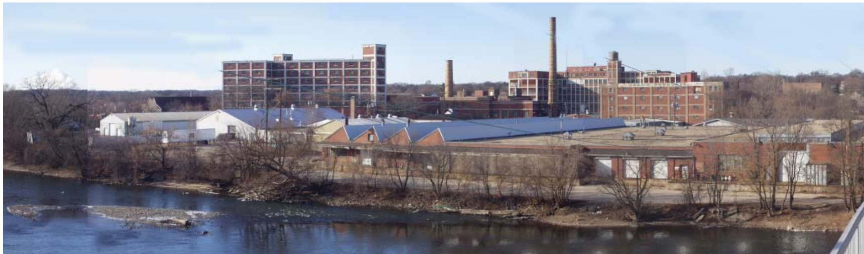
Figure 7.12. View of site overlooking Rock River from Morgan Street bridge.
