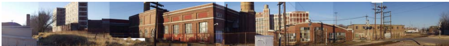
Figure 7.15. Backside view along railroad tracks standing on Loomis Street facing southwest.
