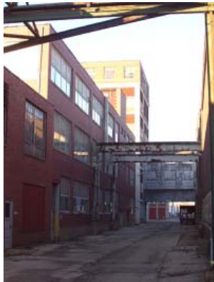
Figure 7.25. Building façade facing east (left); façade facing west (right).
