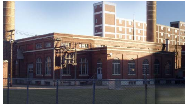
Figure 7.32. Power plant façade facing west.
