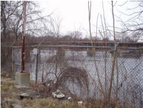
Figure 7.18. View along riverbank facing railroad bridge.
