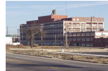
Figure 7.26. Building façade facing east (top); façade facing west (bottom).
