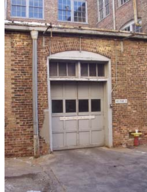
Figure 7.21. Several garage doors of different sizes located throughout site.
