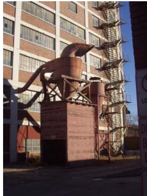
Figure 7.20. Unique exhaust fan serves as focal point.
