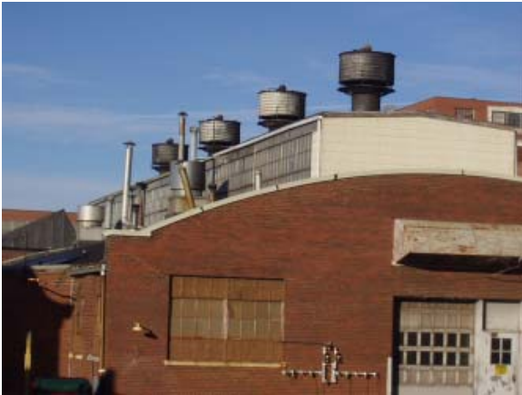
Figure 7.16. Various exhaust fans throughout site.
