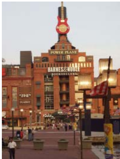
Figure 3.2. Renovated powerplant along Pratt Street- Harborplace- Baltimore, Maryland.
