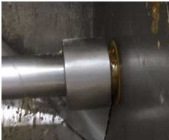
Pic.7 Shaft & Groove Before Cleaning
