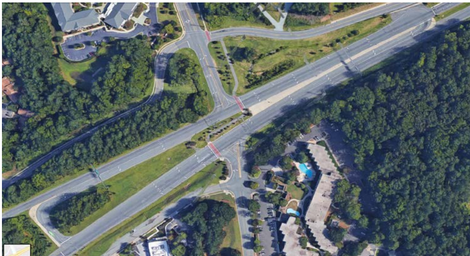
Figure 3. Photo. Example of median U-Turn intersection in Chapel Hill, NC. (10)
