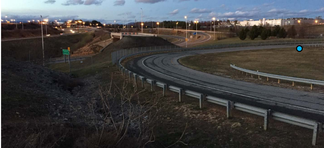
Figure 16. Photo. Roadway lighting adjacent to curve sign.
