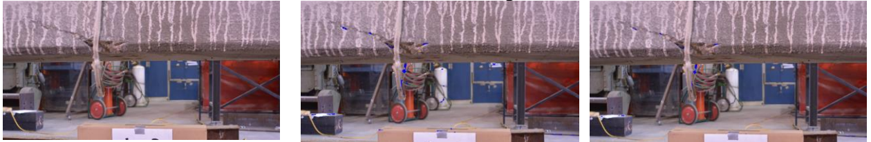
f) Crack on Bottom Flange of I-Beam 9
