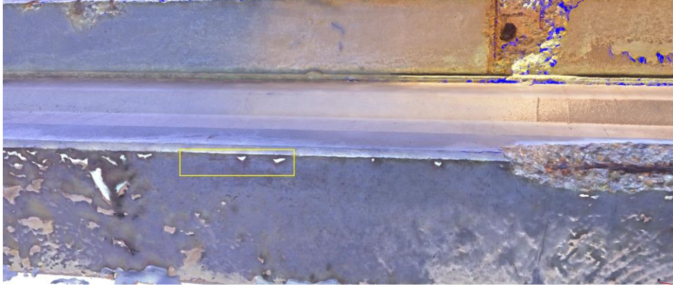
c) Undetected Crack (Bottom)
