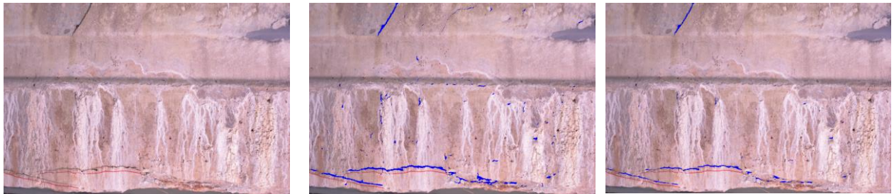
a) Cracks on Side of Box Beam-3
