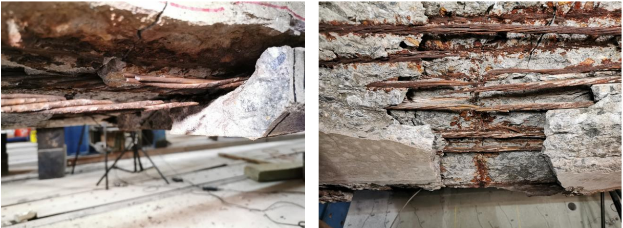
Figure 3.22. Strand Rupture in Test-2 on Aden Road Bridge Box Beam-3
