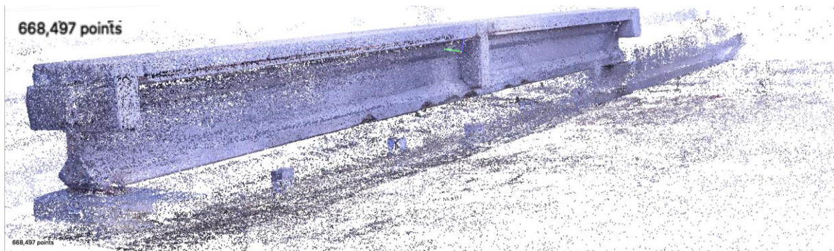
a) Sparse Point Cloud for Lesner Bridge I-Beam 5
