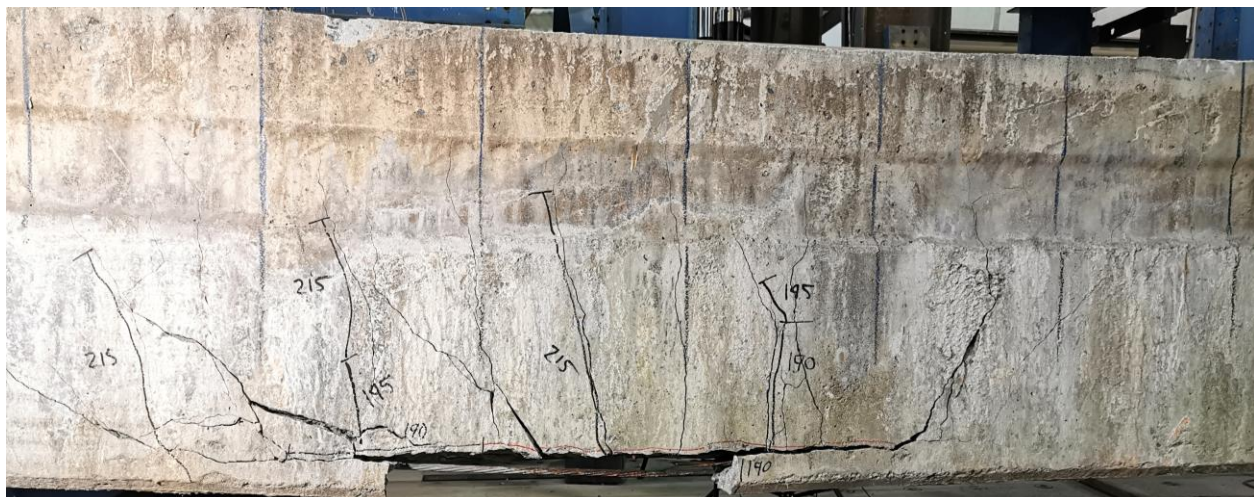
Figure 4.34. Region of Failure in Test-2 on Box Beam-3 from Al Rufaydah (2020)
