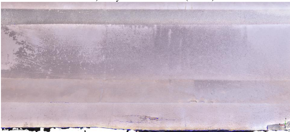
b) Fully Detected Cracks (Side-a)
