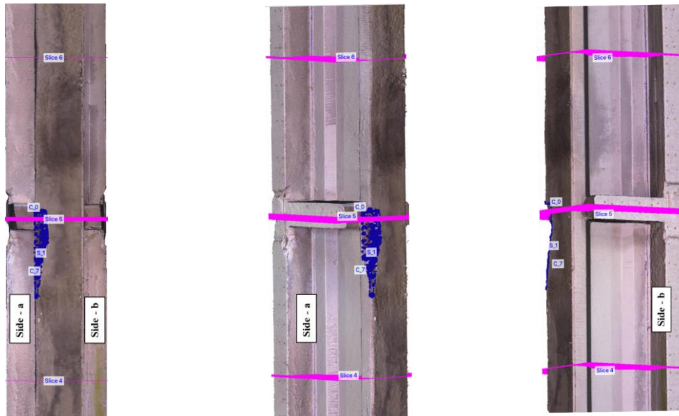
Figure B.12. Damage Clusters in the IW considered for Strength Estimation at Slice-5
