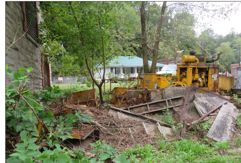
Immediate areas surrounding the building are cluttered with old mining equipment and sometimes overgrown with vegetation, unfortunately making the building unsightly from the street.
