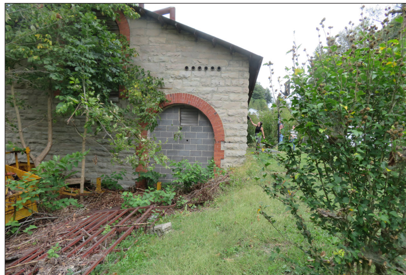
The building is partially built into the former rail bed. Some original pipes remain through the wall.
