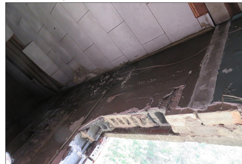
The existing sliding garage door opening is unfinished. The exposed CMU block indicates that this northwest wall is not original.
