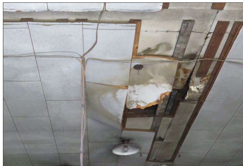
Drop-down ceiling is in poor condition and shows signs of water damage.
