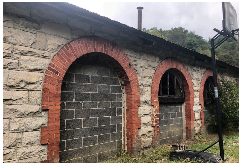
Each original window opening has a striking brick trim. The southeast facade is partially built into the former rail bed.
