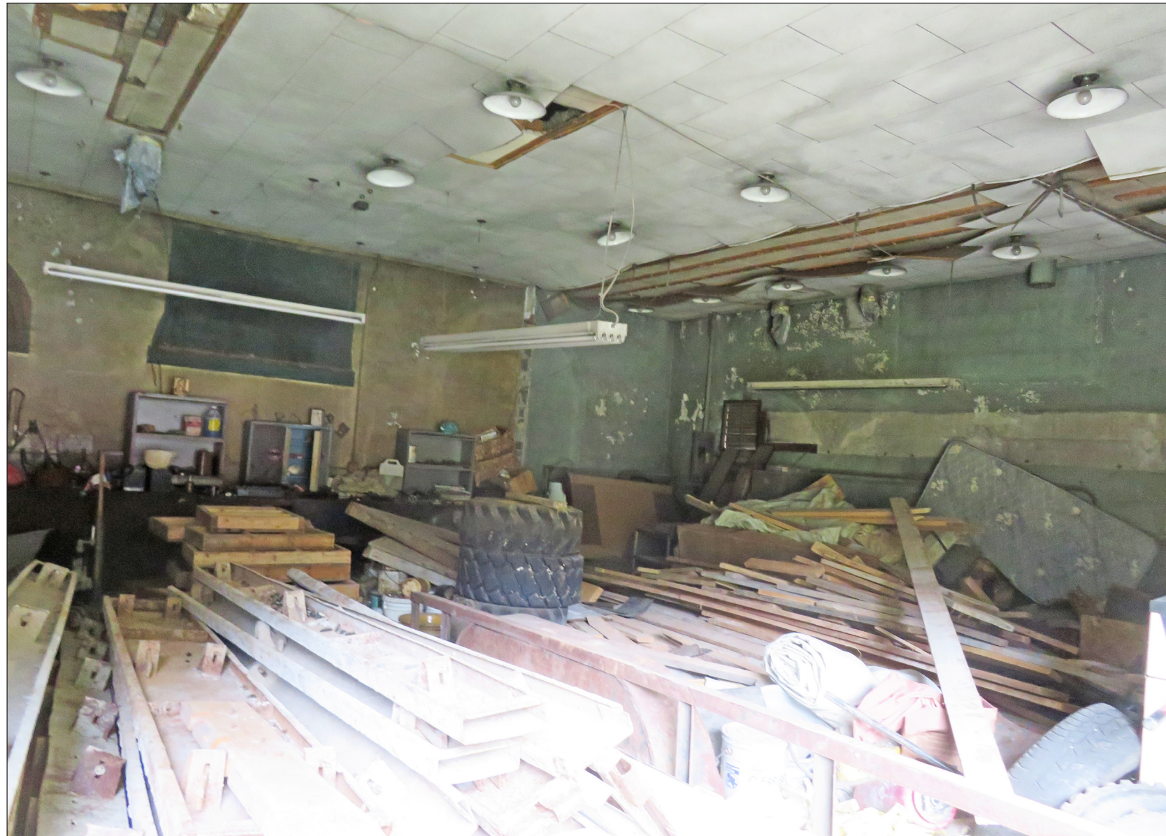
The Steam Building's interior is in moderate to poor condition. The storage of materials inside the building makes it difficult to inspect all portions of the building. Original window openings along the back and side walls have been blocked in and few original ornamentation remains.
