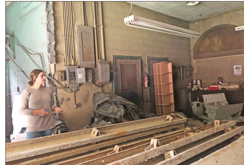
Mechanical panels are disorganized with several wires exposed and unprotected. A bathroom is located behind one of the doors in the middle of the picture.
