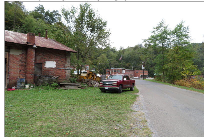
The building sits particularly close to Lower Bearallow Road. Special considerations should be given to pedestrian safety as redevelopment ideas are prepared.
