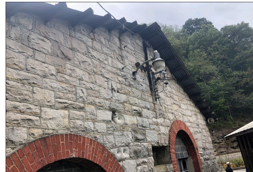
The roof is constructed from simple tin. The unique stonework is an important historical feature of the building.
