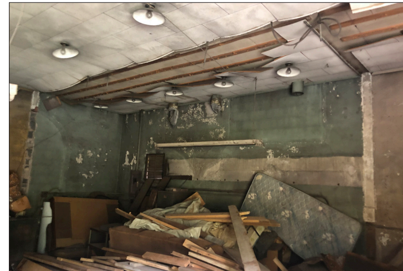
Indicated by the vertical white line on the right hand side, the northwest portion of the building an addition and not original. The drop-down ceiling makes it difficult to see the condition of the attic.
