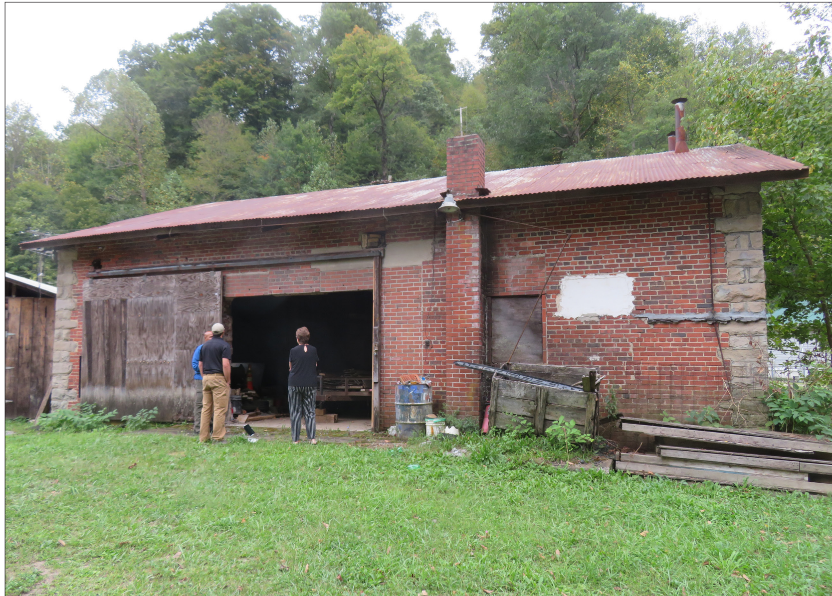
The northwest facade of the Steam Building is primarily brick with decorative stone corners. This facade is an addition to the original structure. A large sliding door to the left of the chimney is the primary access to the building's interior. The property has a secondary storage structure made of wood that can be seen on the far left of the picture above.
