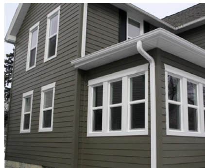
Fiber Cement Siding
