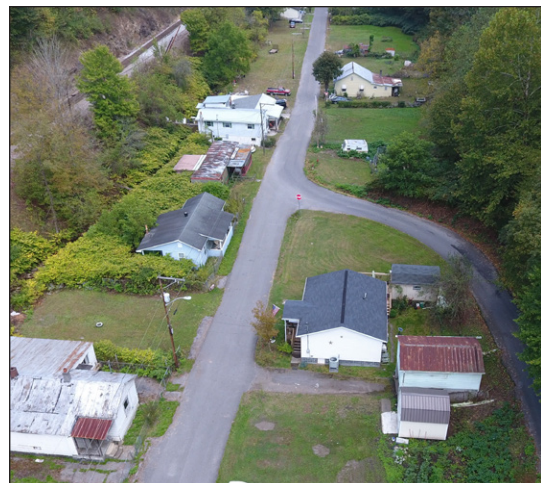
Aerial of Sawmill Hollow (2019)
