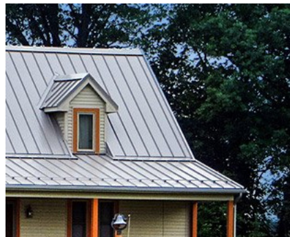
Standing Seam Metal Roof
