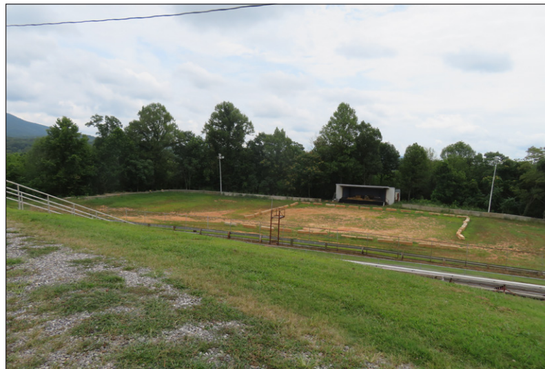
Looking down the slope toward the demolition derby area. The structure in the middle has fallen into disrepair and needs improvements.
