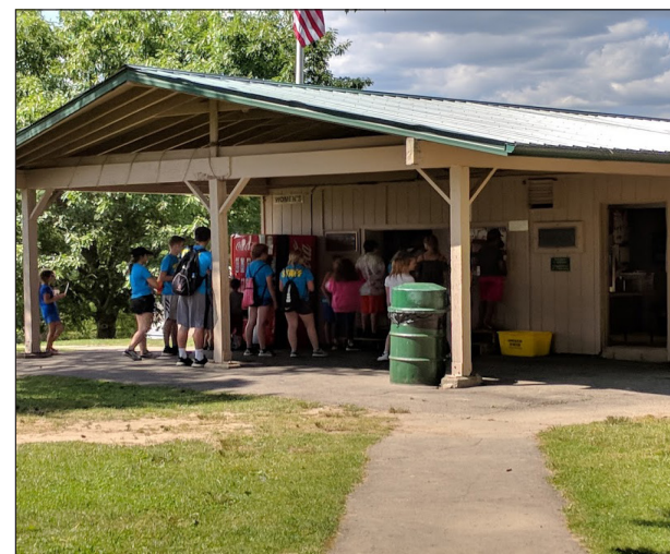
A combined concession/restroom building with covered areas to gather.
