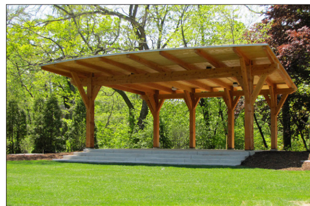
The stage is a timber frame and open air design.
