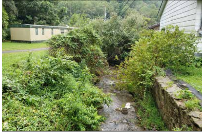
5: A retaining wall separates Mill Creek from the playground and basketball court. While there is seldom flooding from water level rise, poor drainage infrastructure throughout the town can cause flooding.
