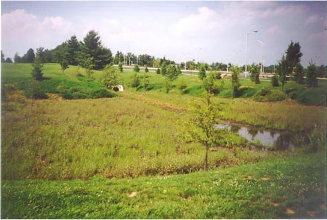
Figure 3-7. Pond with Grass Cover and Low Flow Channel
