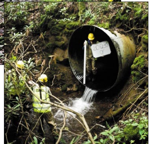
Pipes with significant drops can block many fish from passing upstream.
