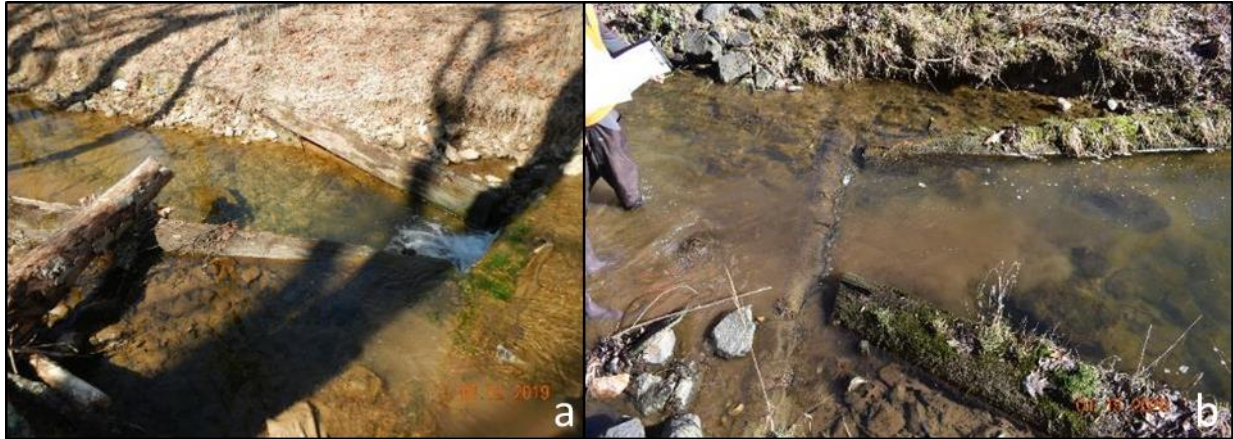
Figure 3.8 Two examples of log full span vanes from restoration projects 28 (a) and 36 (b).
