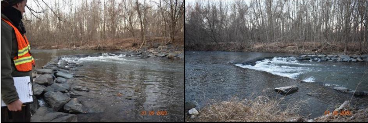
Figure 3.7 A cross vane constructed using dumped stone from restoration project 35.
