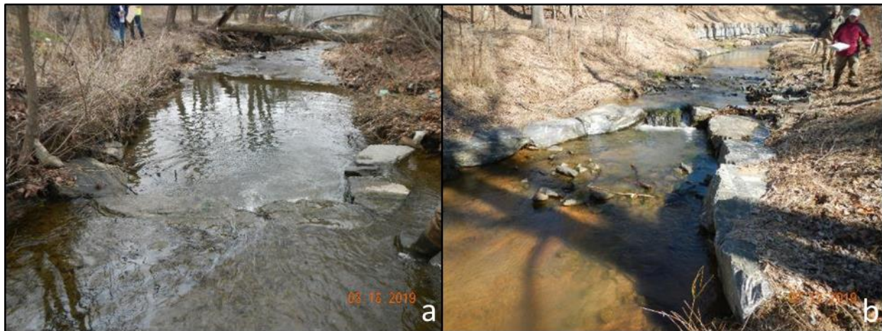
Figure 3.9 Two examples of rock full span vanes from restoration projects 24 (a) and 28 (a).
