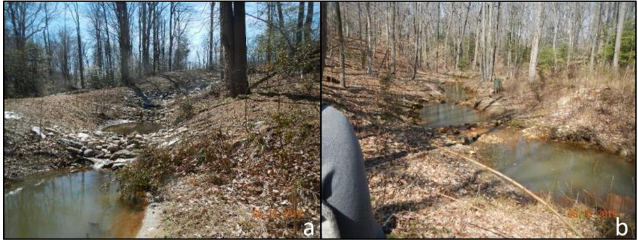
Figure 3.25 A high gradient regenerative stream conveyance (RSC) structure at restoration project 6 (a) and a low gradient RSC sequence at restoration project 6 (b).
