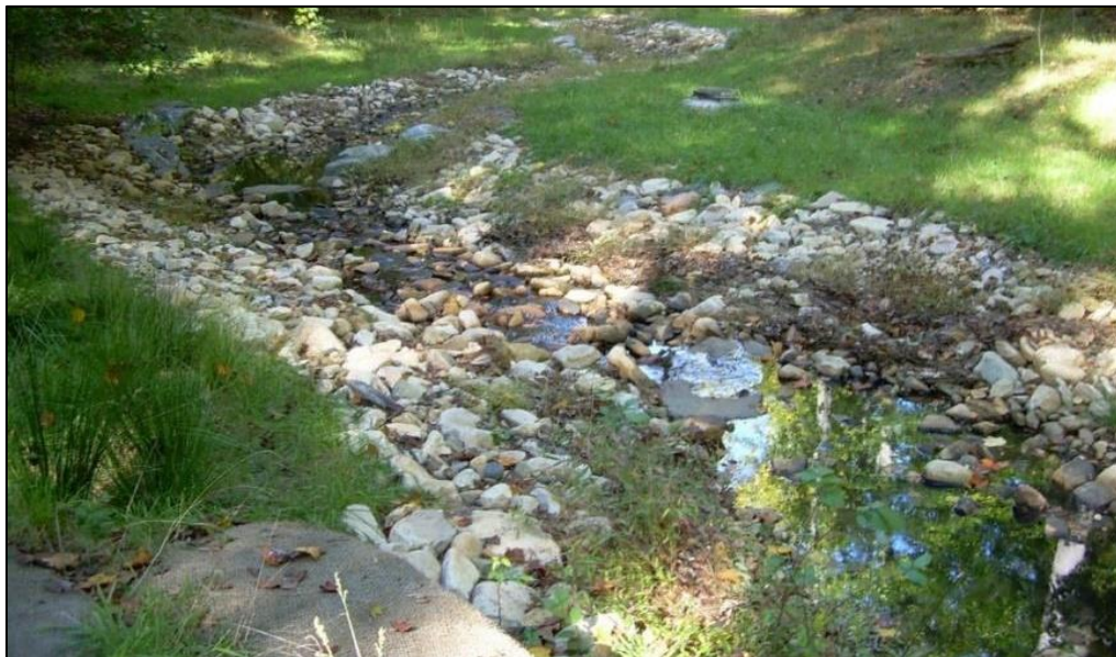
Figure 3.63 Example of unstacked BP from an unassessed restoration project in Maryland.
