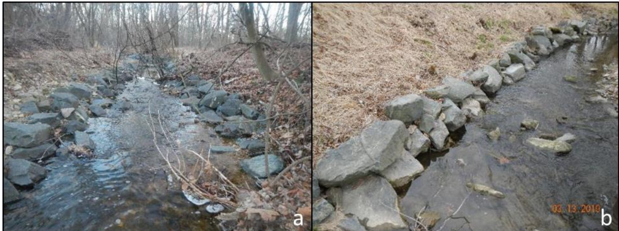
Figure 3.4 Examples of stone toe from restoration project 22 (a) and 33 (b).
