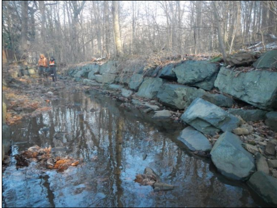
Figure 3.37 Stacked imbricated bank protection from restoration project 2.
