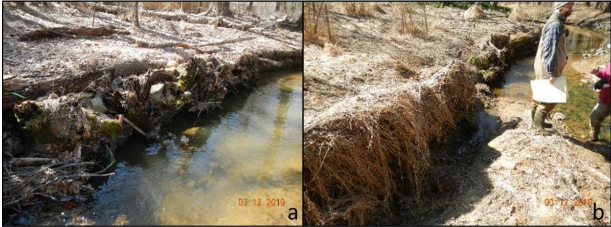
Figure 3.35 Pictures of log meander protection from restoration project 28.
