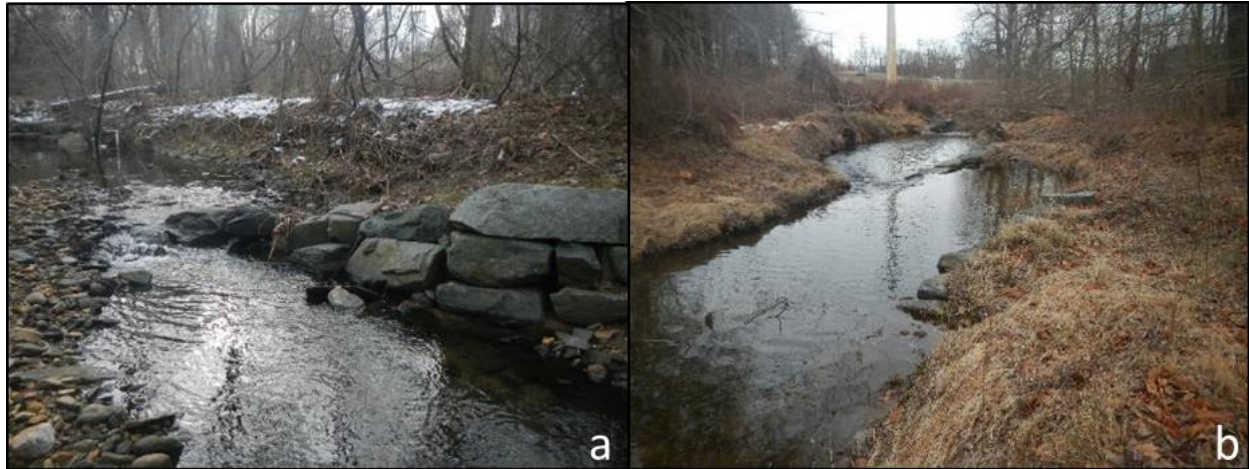
Figure 3.14 Two examples of rock partial span vanes. A single arm vane from restoration project 7 (a) and two single arm vanes from restoration project 31 (b).
