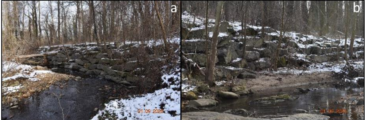
Figure 3.61 Examples of stacked bank protection from restoration project 16.
