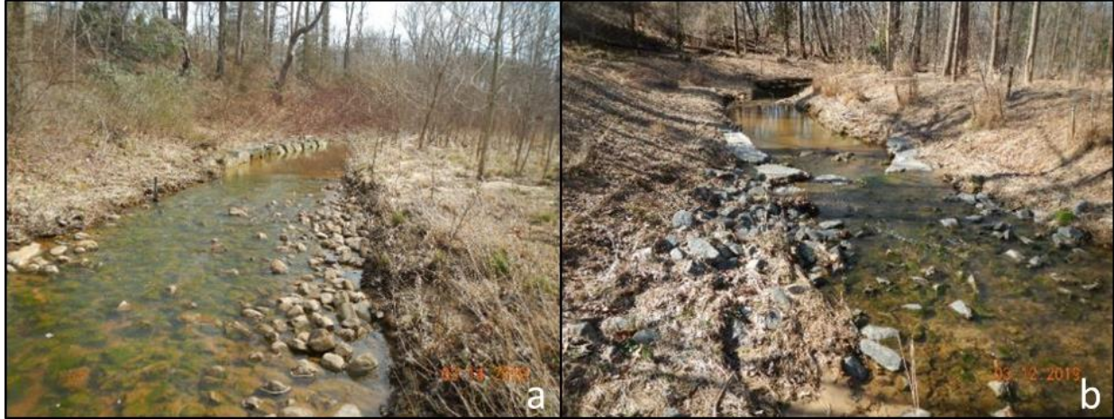
Figure 3.22 Two examples of RFs that did not utilize armor on the adjacent banks. Constructed riffle from restoration project 9 (a). Constructed riffle from restoration project 28 that is constructed directly upstream of a cross vane that is providing stabilization (b).
