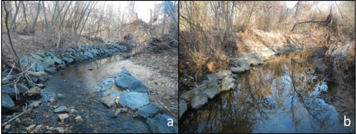
Figure 3.64 Examples of unstacked bank protection from restoration project 22.
