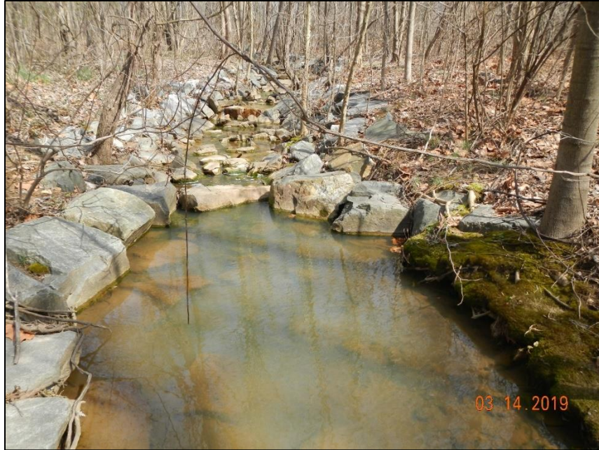
Figure 2.11 Conservative design of project 19 used large rock relative the channel size.
