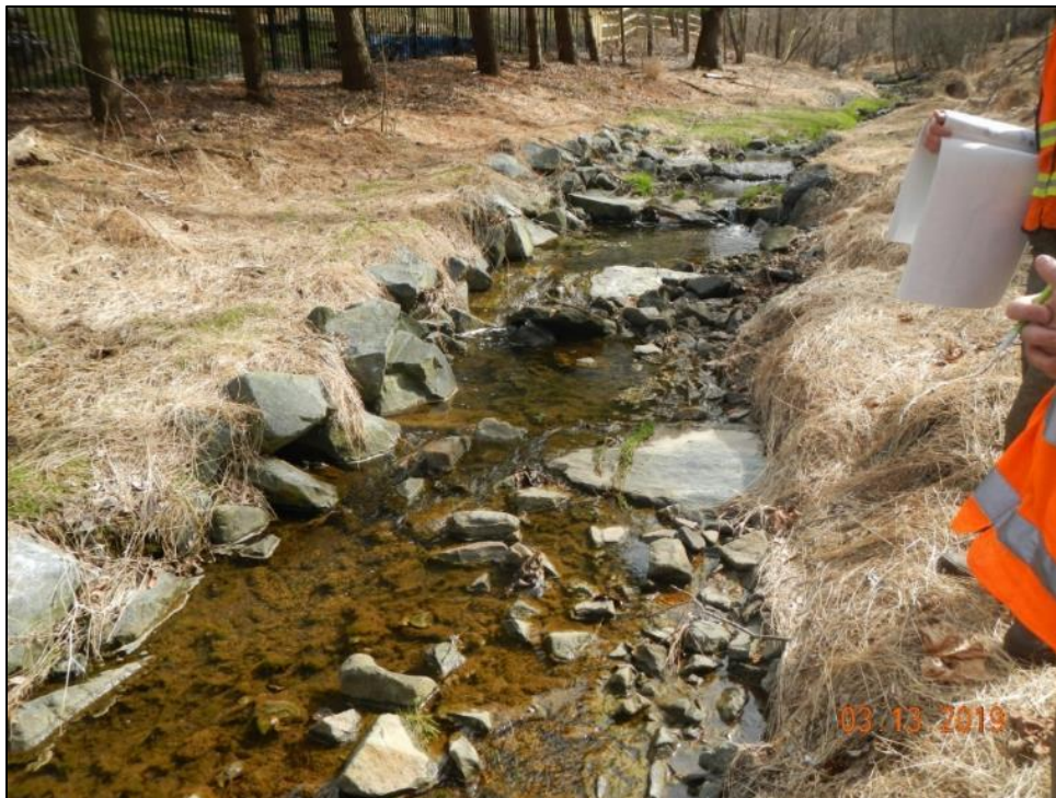
Figure 3.38 Unstacked bank protection from restoration project 3.
