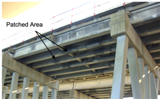
Figure 5.2. Typical Deterioration on the Lesner Bridge (left) Cross-section of Lesner Bridge I-Beams (Right)
