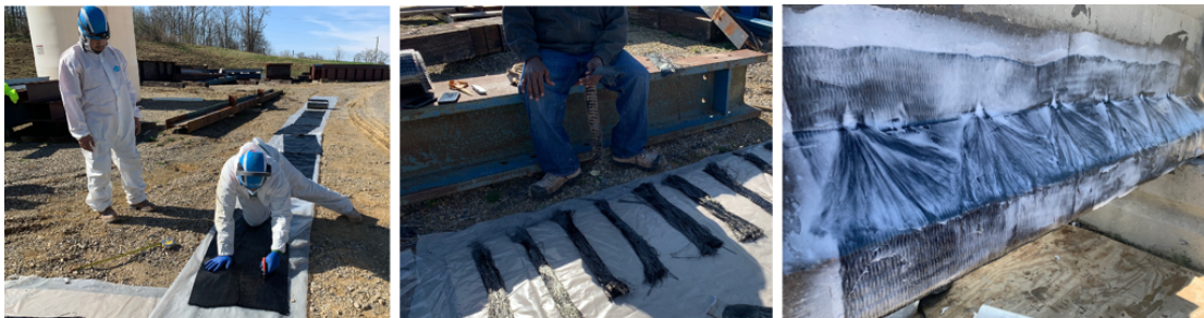
Figure 5.11. CFRP Installation on I- Beams
