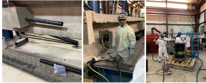
Figure 4.8. External Post-Tensioning Repair
