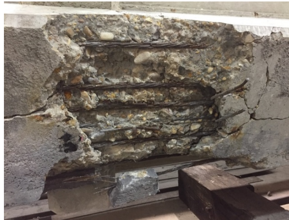
Figure 3.7. Bottom Flange of I-Beam 2 after Testing
