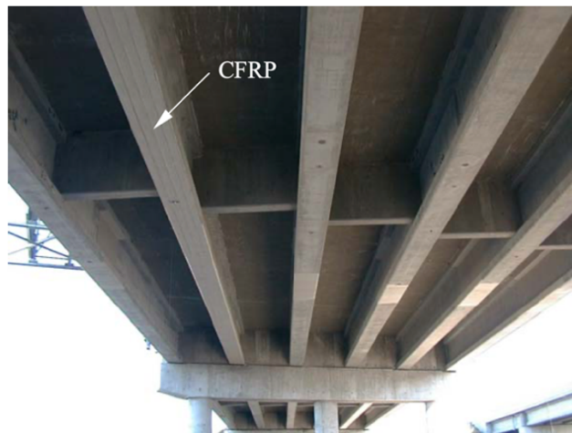
Figure 2.18. CFRP sheets attached to the repaired beam
