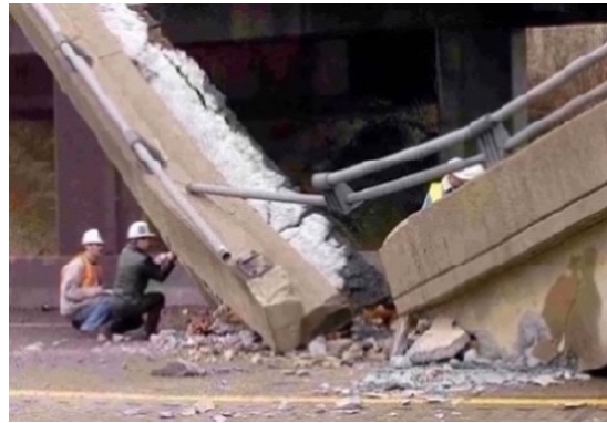
Figure 2.2. Collapse of Lake View Drive Bridge
