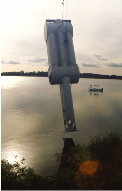
Figure 1. Photograph of full-lift aerator prior to installation. (Photo from Bob Kortmann of Ecosystem Consulting Service, Inc., used with permission.)
