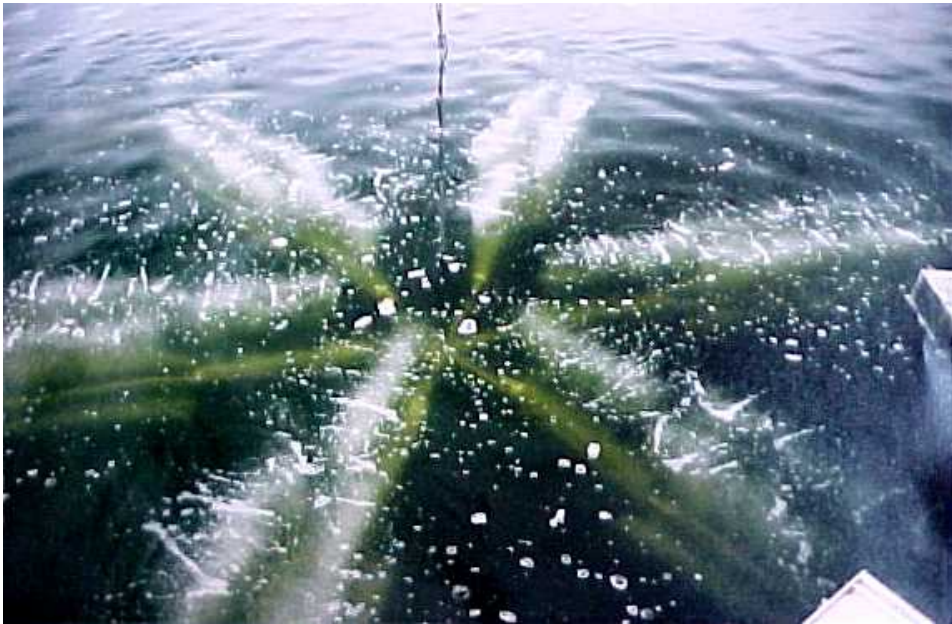
Figure 3. Photographs of linear (top) and circular (bottom) bubble-plume diffusers. (Photo of linear diffuser from Mark Mobley of Mobley Engineering, Inc. Photo of circular diffuser from Swiss Federal Institute for Aquatic Science and Technology. Both photos used with permission.)
