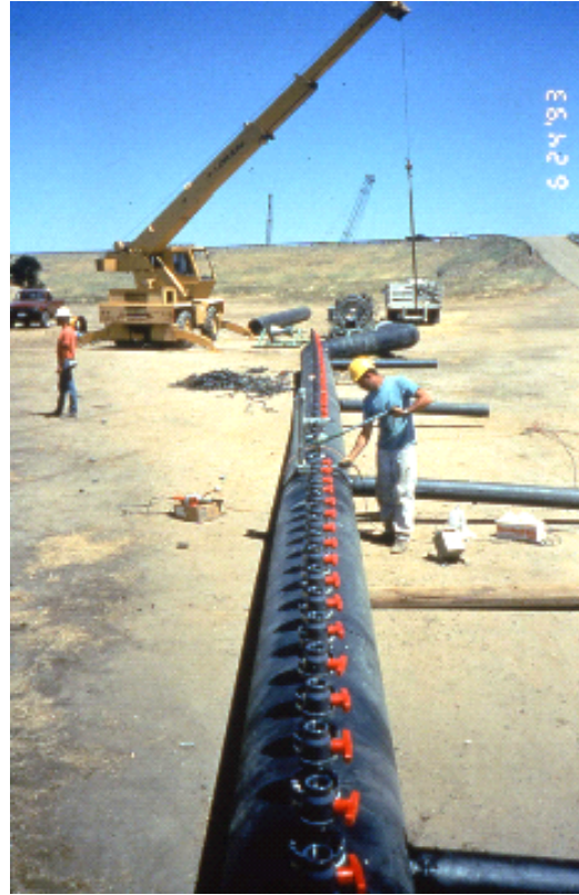
Figure 2. Photographs of Speece Cone and diffuser prior to installation at Camanche Reservoir, California. (Photos from Rod Jung of East Bay Municipal Utility District., used with permission.)
