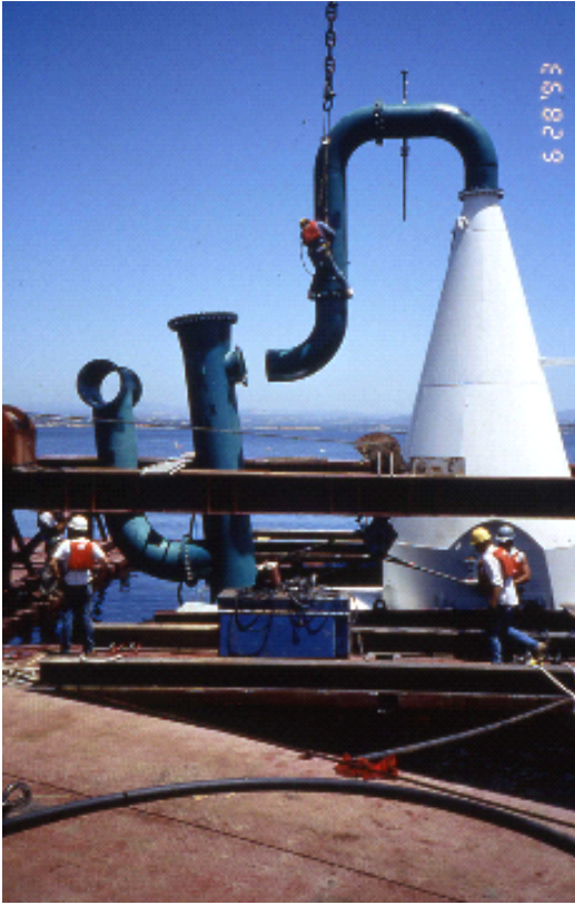
Figure 2. Photographs of Speece Cone and diffuser prior to installation at Camanche Reservoir, California. (Photos from Rod Jung of East Bay Municipal Utility District., used with permission.)
