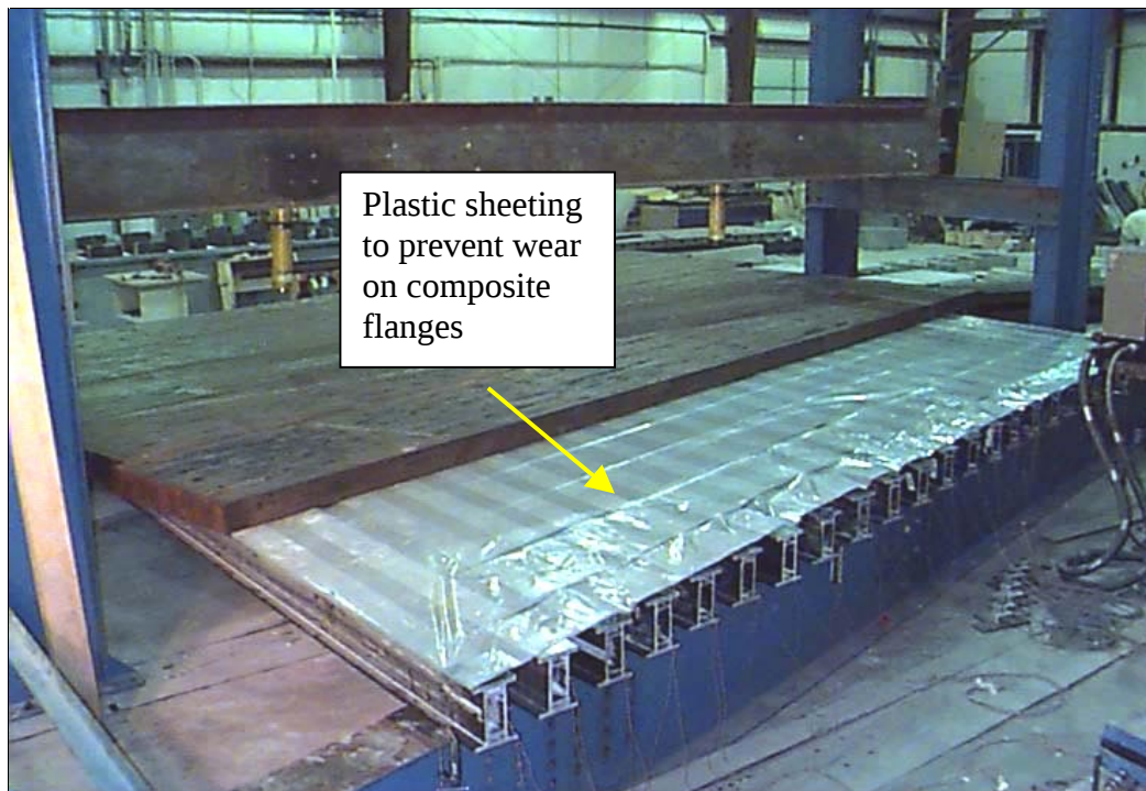
Figure 2-7. Assembly of bridge mock-up in the laboratory.
