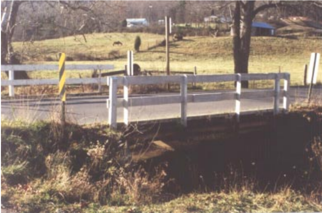
Figure 1-1. Side view of the old Tom's Creek Bridge.
