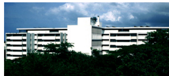
The Women's Dormitory designed by architect Henry Klumb
