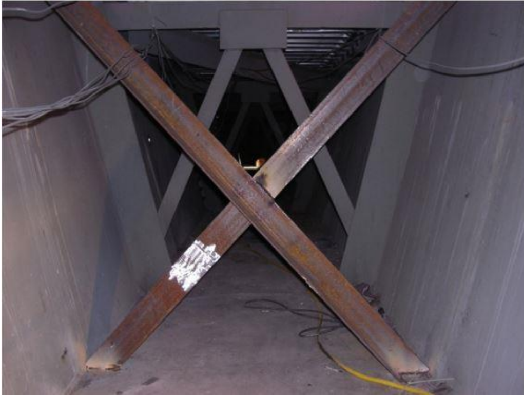
Figure 5-4: Additional cross frame installed inside the exterior girder (Neuman, 2009), used under fair use.
