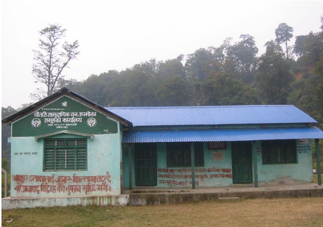
Picture A7.1: Chautari CF Office Building in Background the Forest
