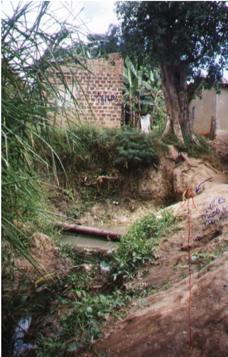
Plate 5: Showing an open spring well found below a toilet.
