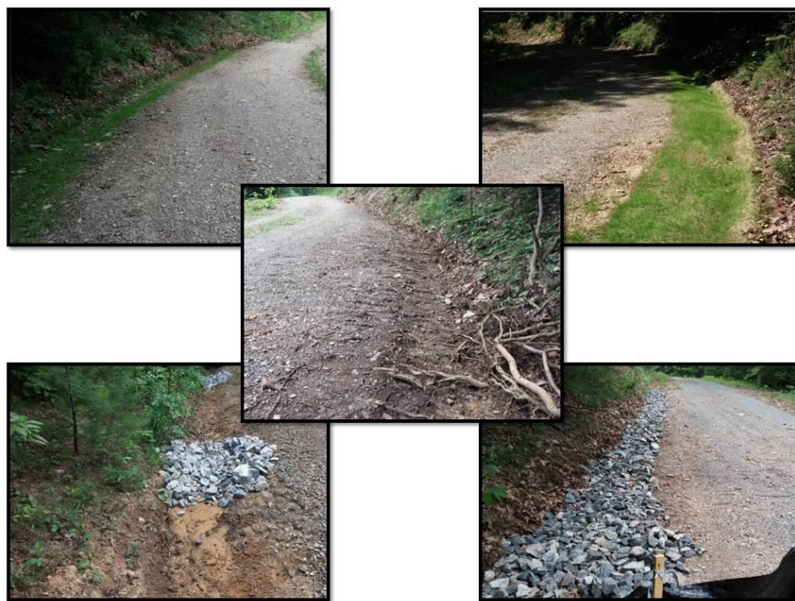
Figure 4.3. Representative ditch best management practices on haul roads stream crossing approaches. Seed (top-left), Mat (top-right), Dam (bottom-left), Rock (bottom-right), and Bare (middle) treatments.
