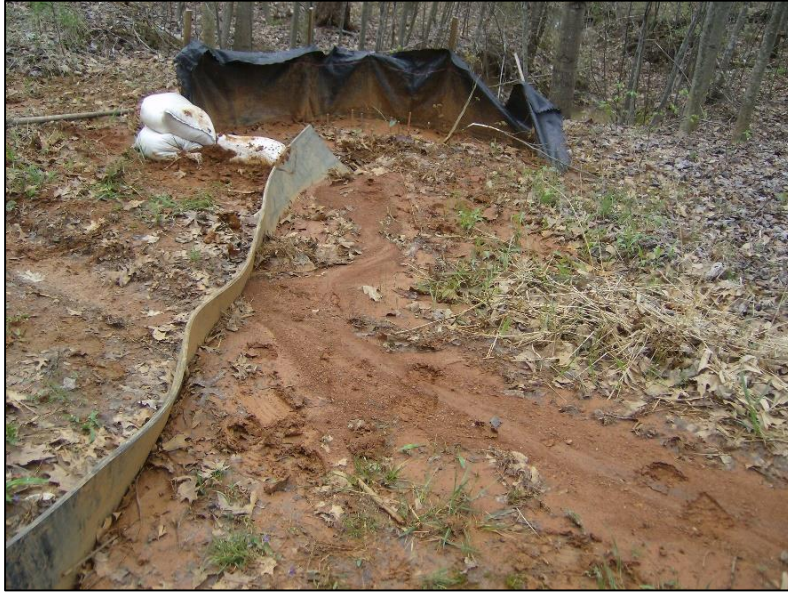
Figure 3.1. Rubber conveyor belt used to divert runoff into silt fence catchment areas.
