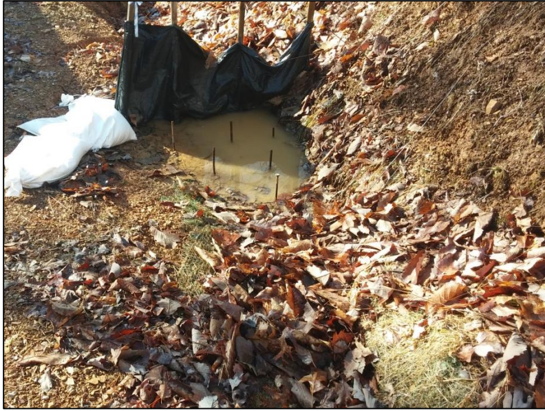
Figure 4.2. Silt fence catchment area with rebar pins marking the location of measurement. Photo taken October 31, 2014 (about five months after study installation).
