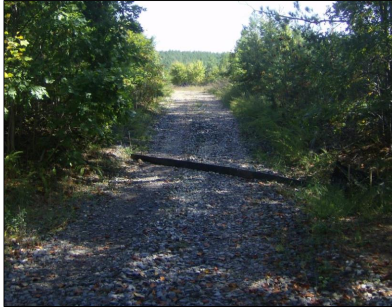
Figure 2.2. Rubber conveyor belt diverter used to divert runoff into silt fence catchment areas.
