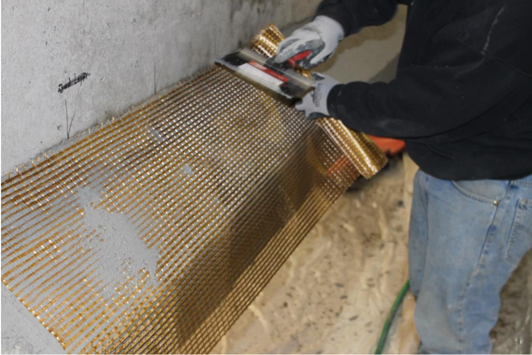
Figure 146- Installation of the First Layer of FRCM Mesh
