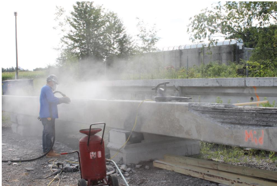
Figure 50- Sandblasting of the Girder Concrete
