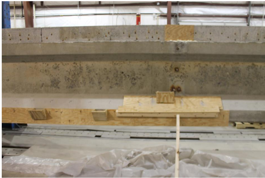
Figure 68- Formwork for the Patch Material
