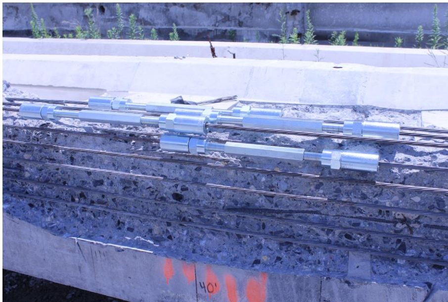
Figure 52- Completed Installation of the Strand Splices
