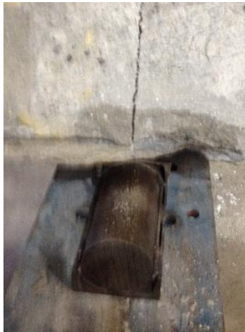
Figure 23- Pin Bearing
