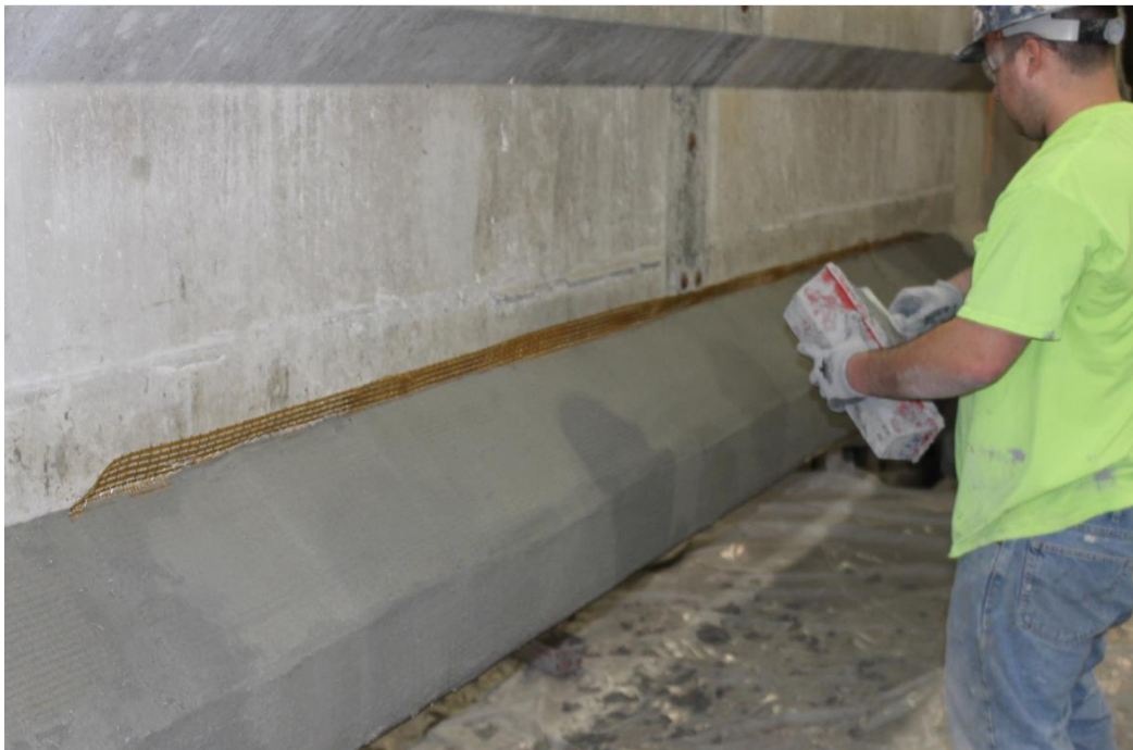
Figure 148- Final Layer of Mortar
