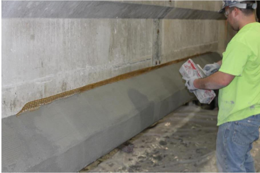
Figure 74- Completed FRCM Repair
