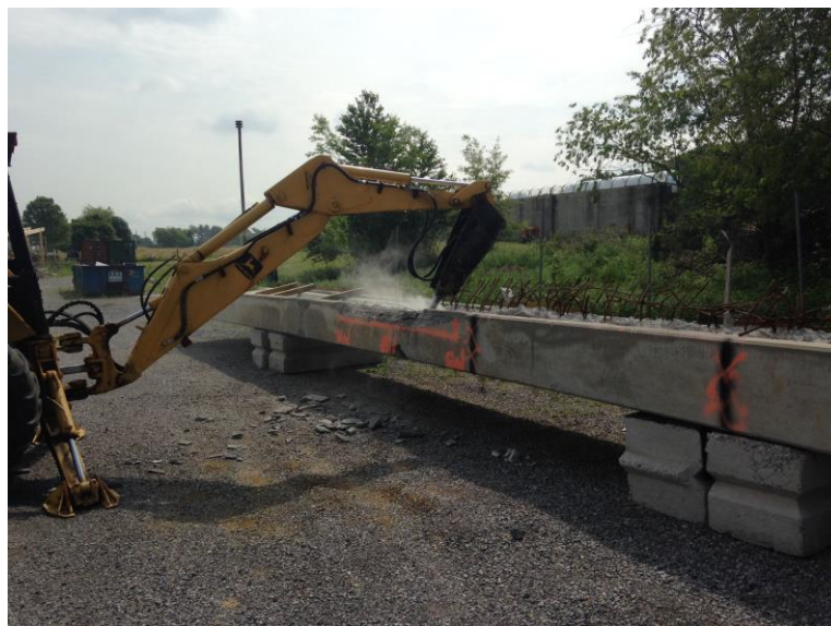
Figure 35- Damaging Girder B with Hydraulic Hammer
