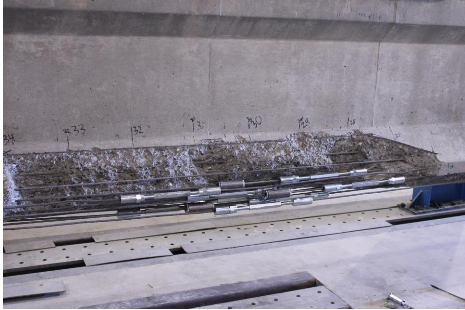
Figure 38- Completed Installation of Strand Splices
