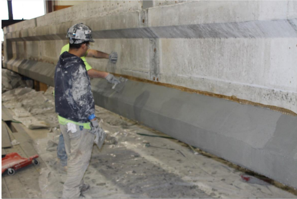
Figure 89- Completed FRCM Repair
