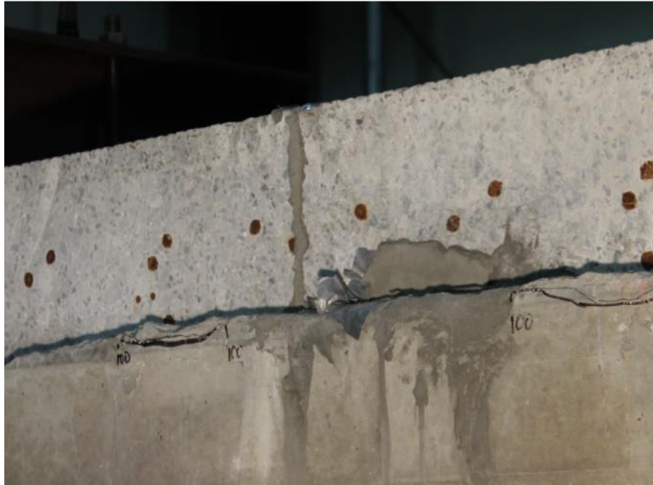
Figure 91- Filling of Saw Cuts in Deck with Grout
