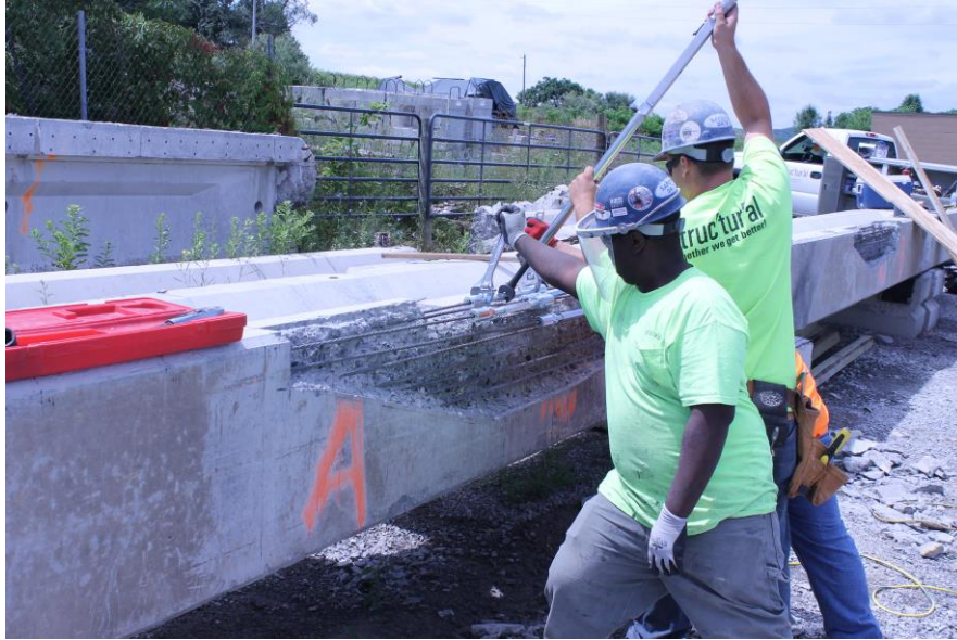
Figure 51- Installation of the Strand Splices
