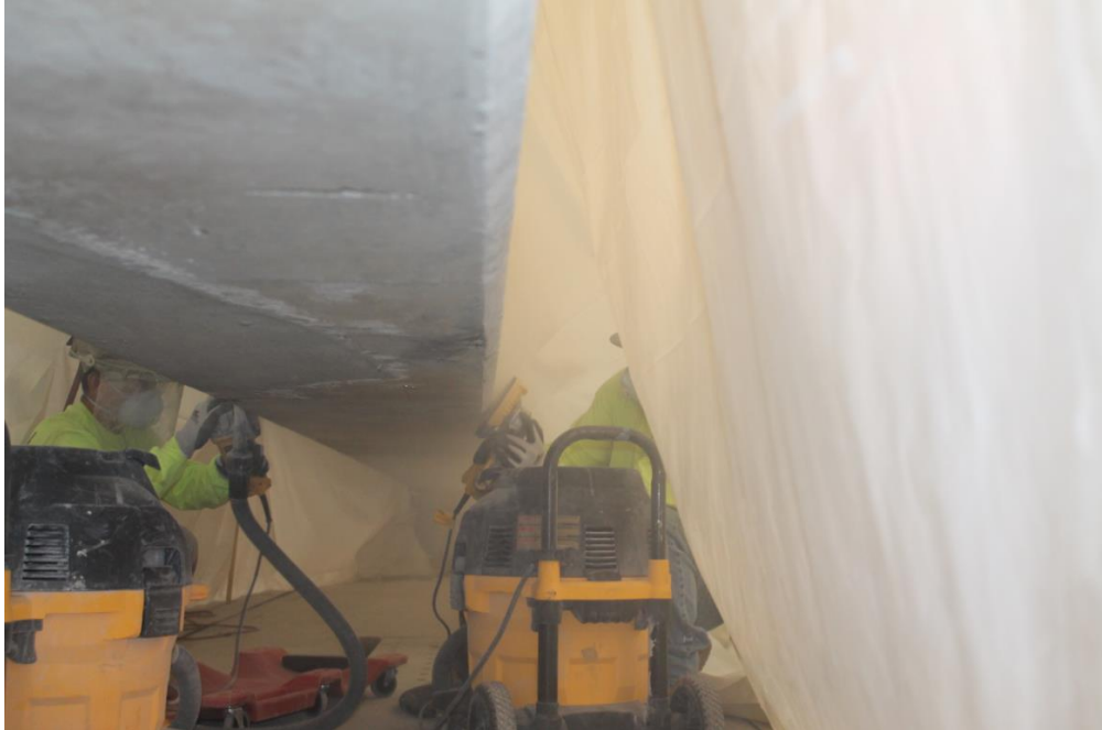
Figure 144- FRCM Surface Preparation using Sanding Wheel
