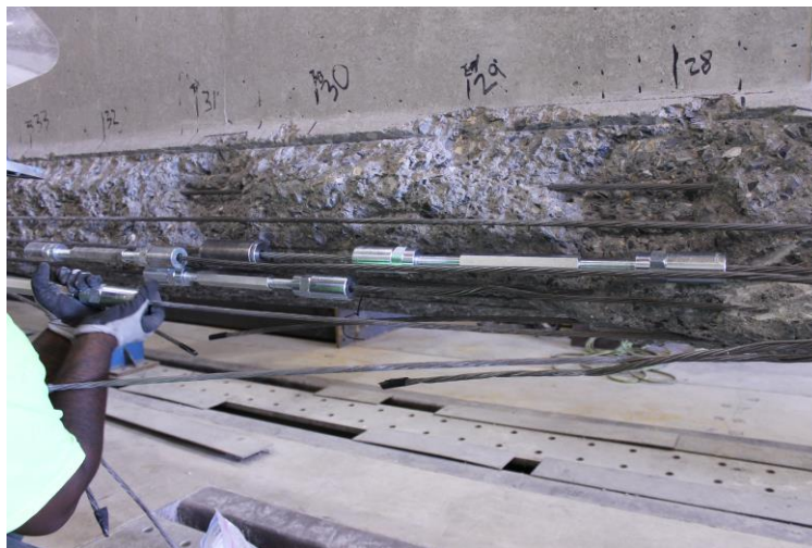
Figure 37- Splice Installation for Girder B Repair
