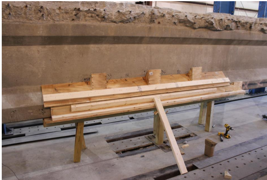
Figure 39- Formwork for Concrete Placement
