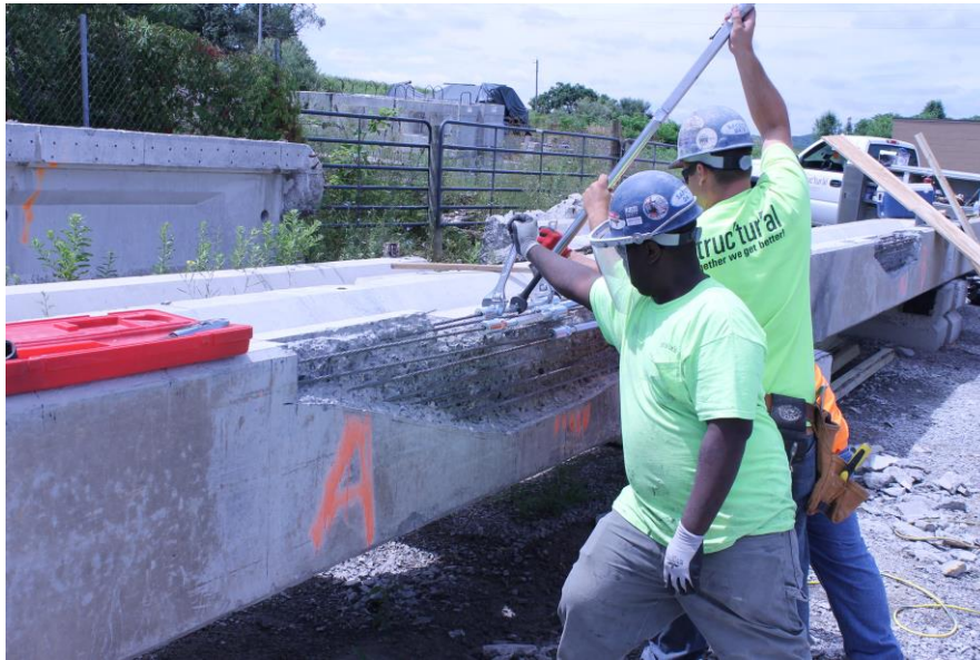
Figure 142- Tensioning of Strand Splice
