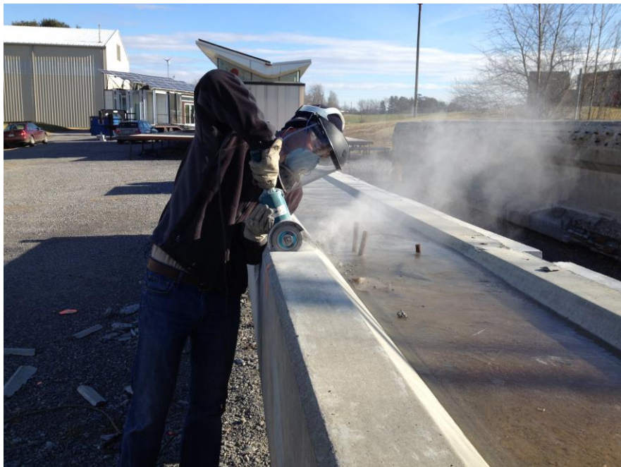
Figure 138- Saw Cutting around Damage Perimeter
