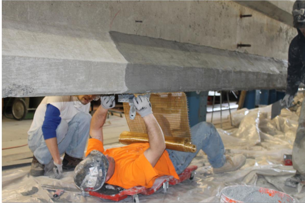
Figure 87- Installation of the First Layer of FRCM Mesh on the Bottom Face
