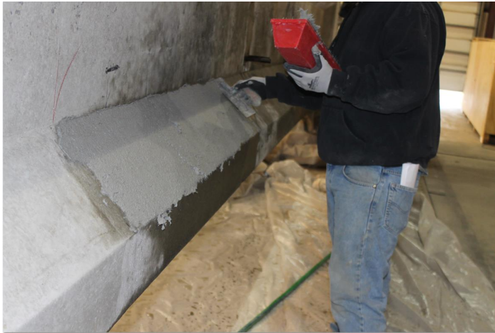
Figure 86- Application of the First Layer of Mortar for FRCM Installation
