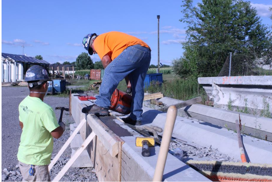
Figure 53- Placing the Repair Concrete
