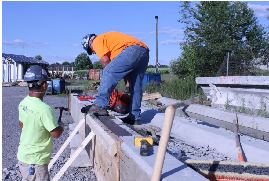
Figure 141- Placing Repair Concrete
