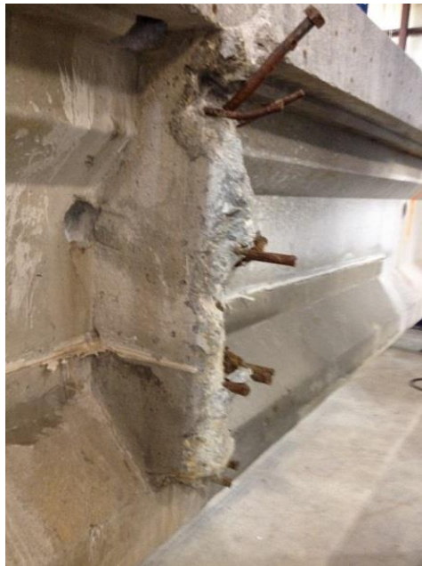
Figure 28- Existing Section of Intermediate Diaphragm
