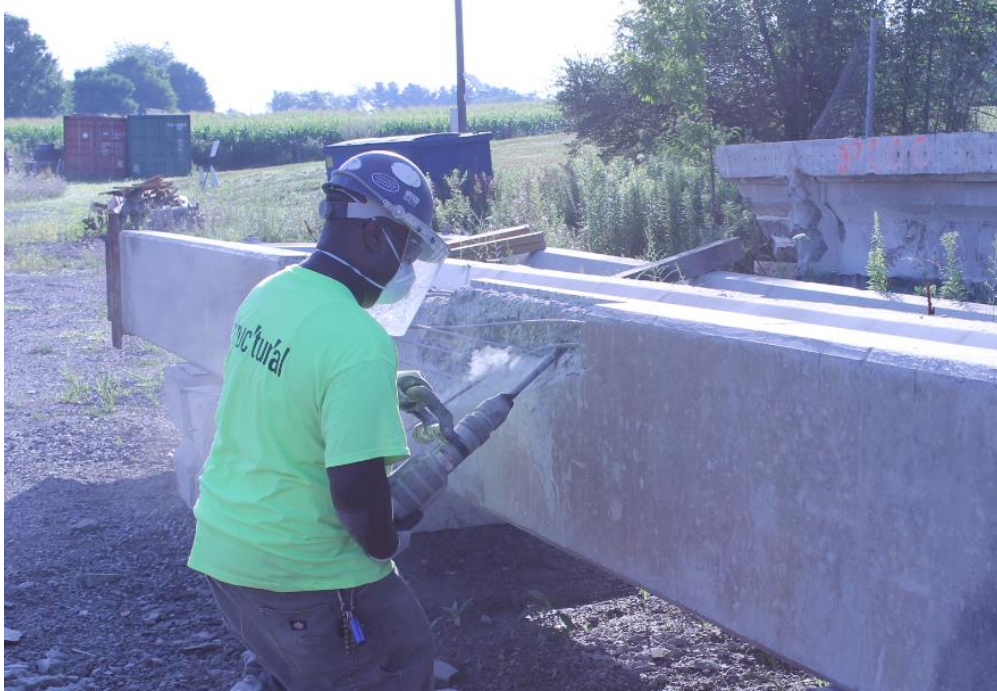
Figure 139- Chipping Concrete with Light Chipping Gun
