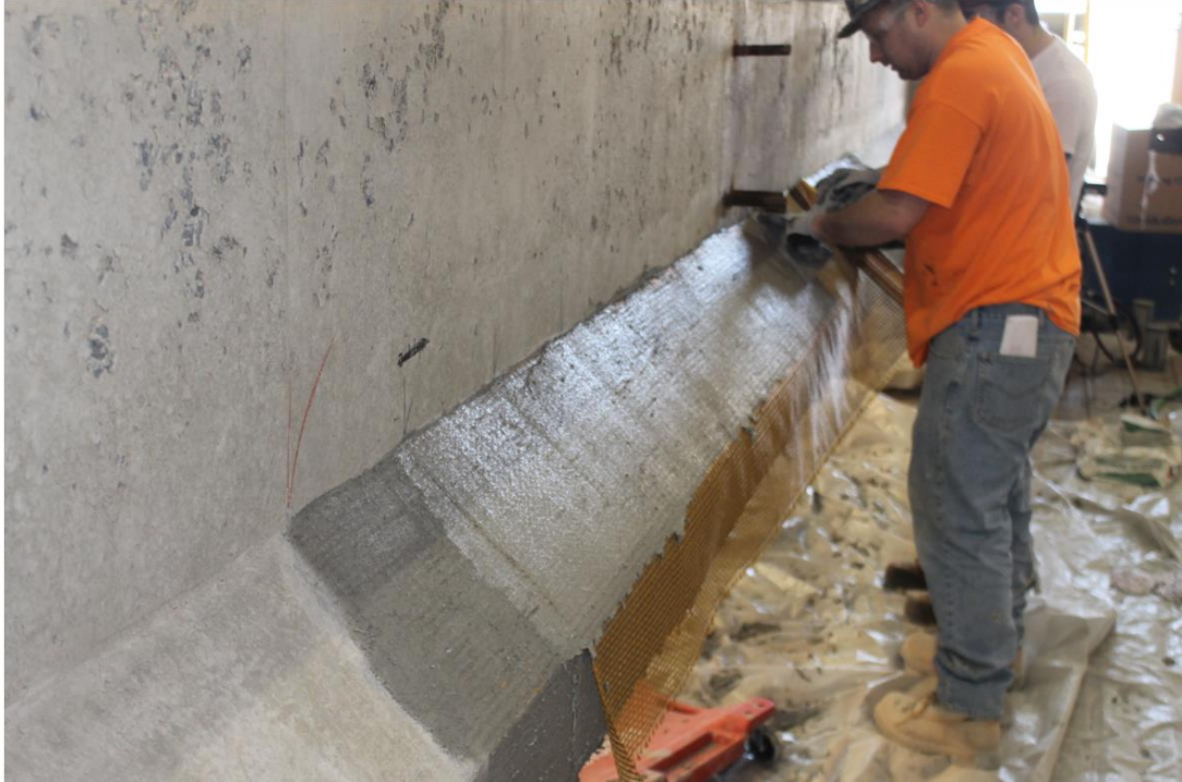
Figure 147- Installation of the Second Layer of FRCM Mesh
