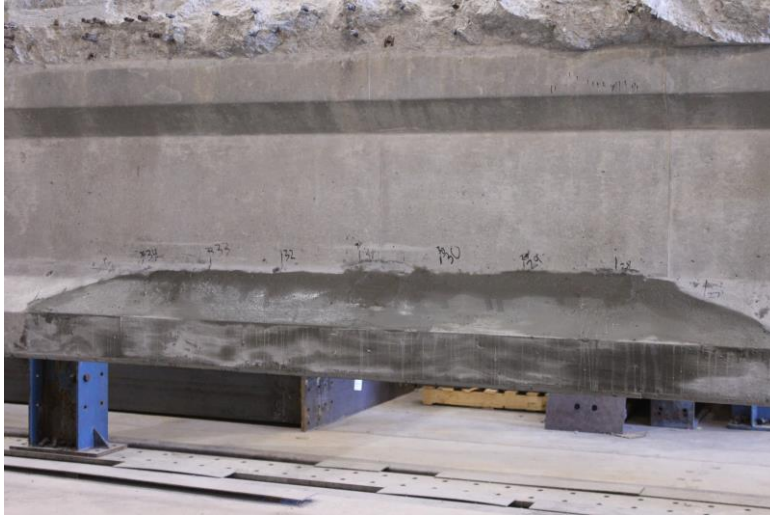
Figure 40- Completed Repair after Concrete Placement and Form Removal
