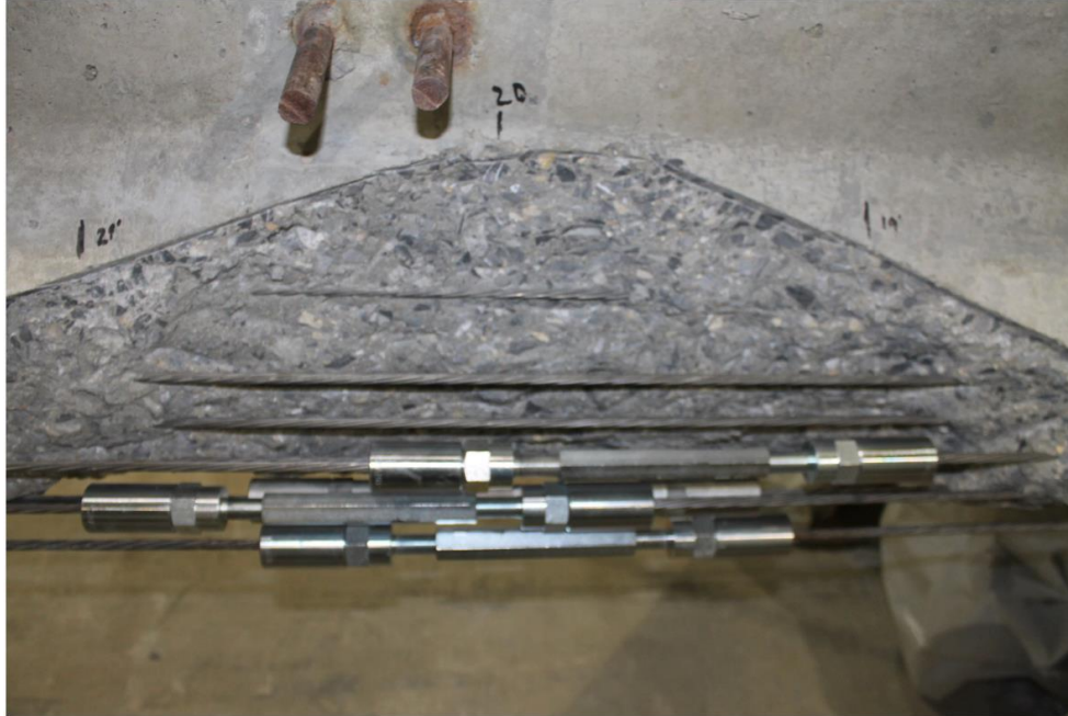
Figure 83- Strand Splice Installation
