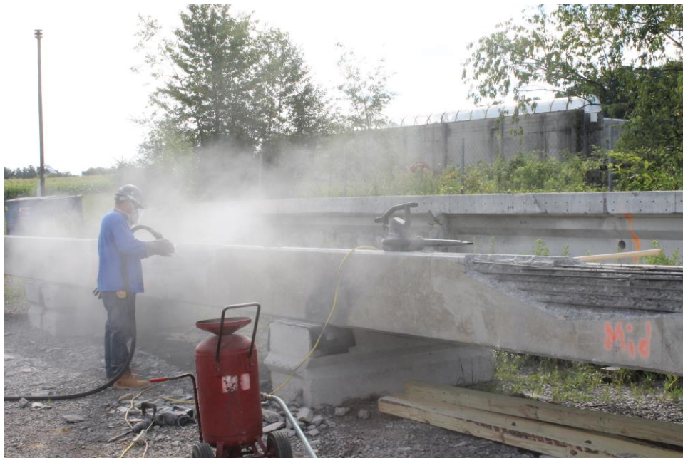
Figure 140- Sand Blasting to Clean Concrete Surface
