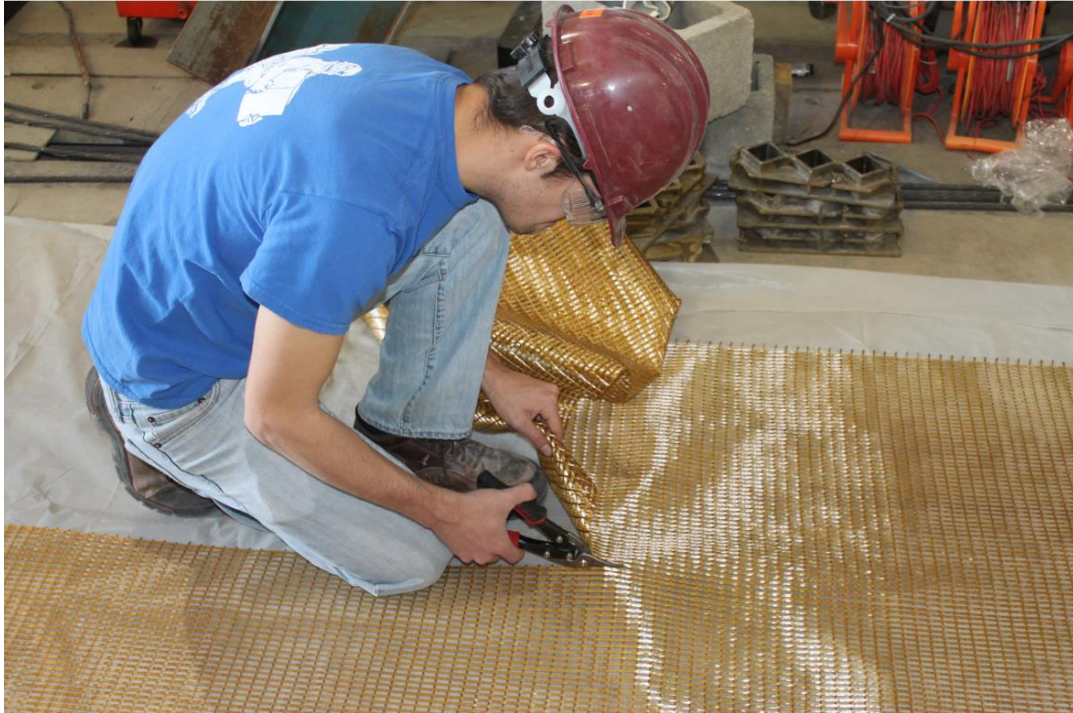
Figure 143- Cutting the FRCM Mesh
