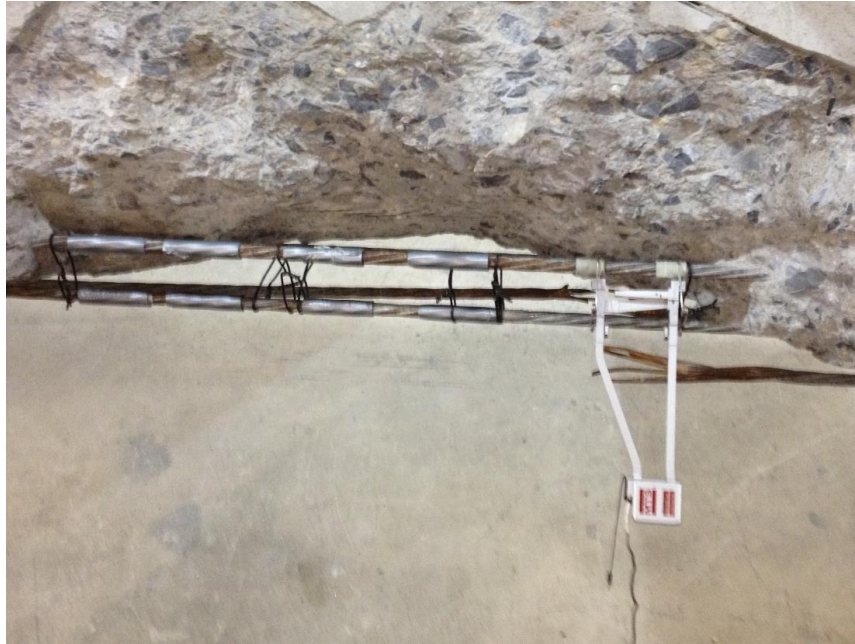
Figure 17- Test Setup to Determine Effective Prestress During Strand Cutting
