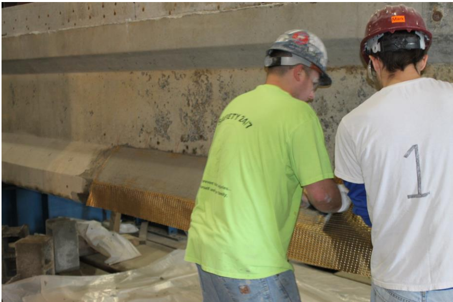
Figure 73- Installation of the FRCM
