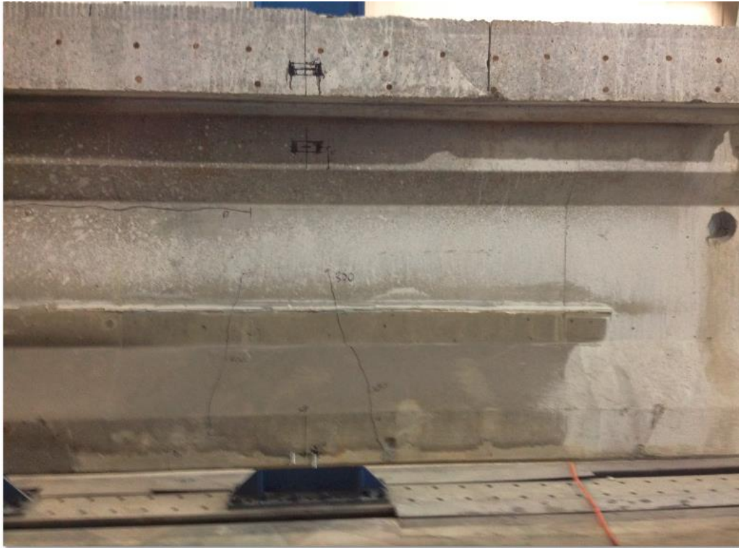
Figure 102- Flexural Cracking in the Bottom Flange and into the Web
