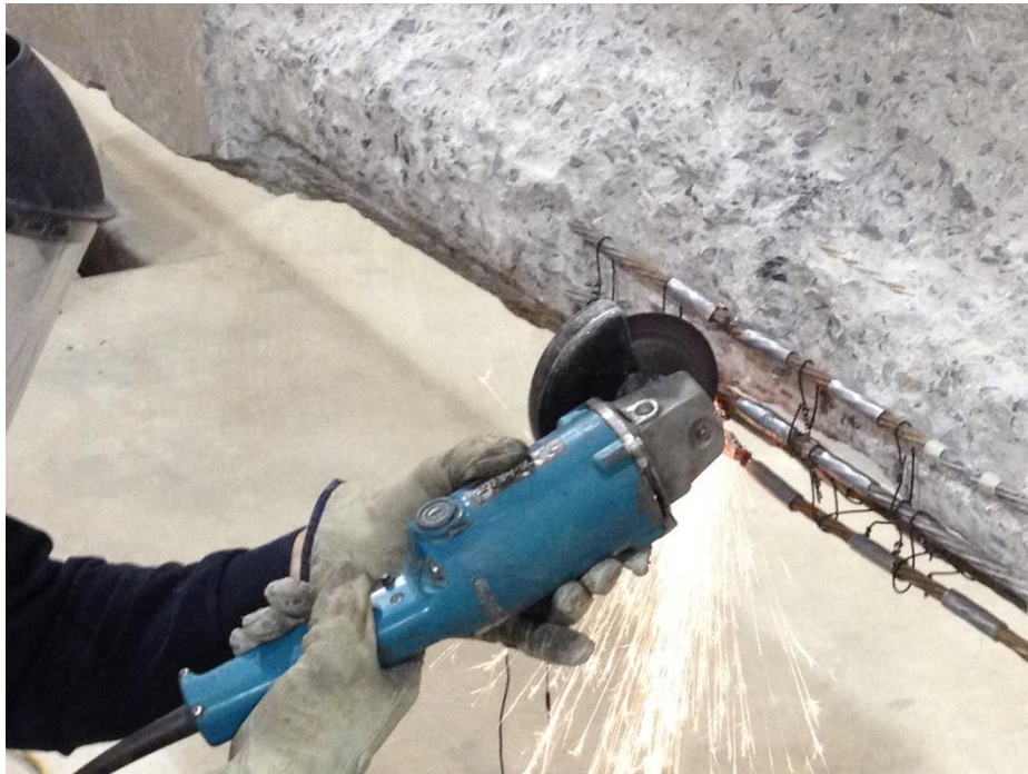
Figure 16- Strand Cutting Using an Electric Grinder
