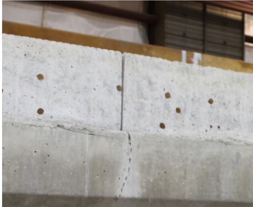
Figure 79- Saw Cut Gaps in the Deck Concrete of Girder D
