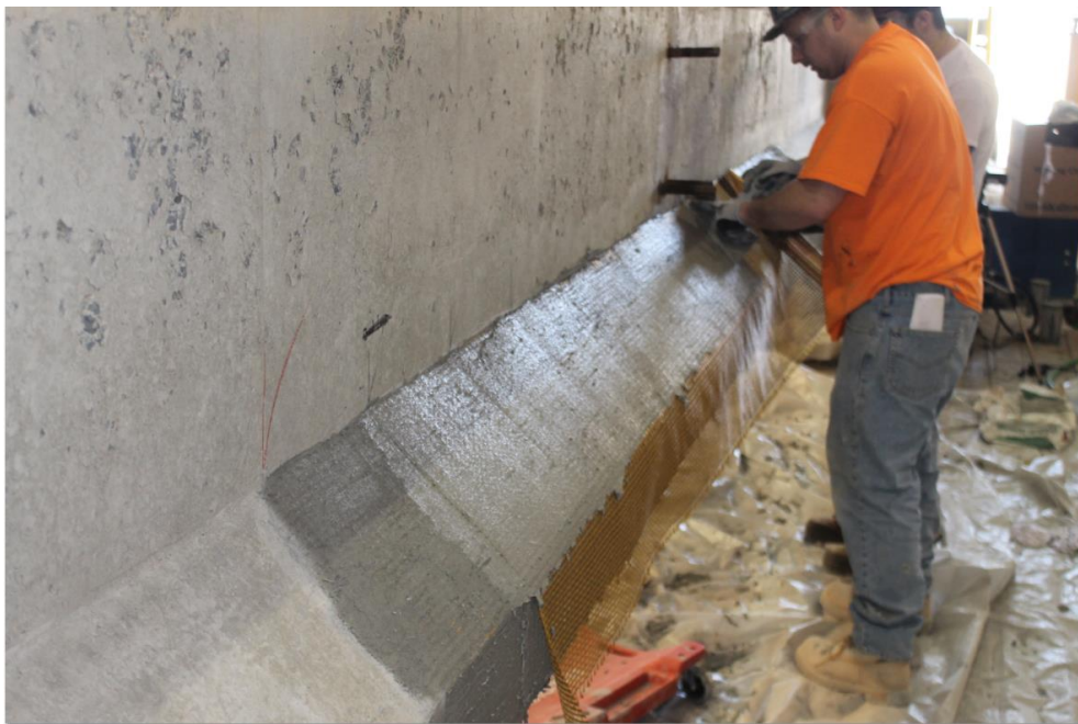
Figure 88- Installation of the Second Layer of FRCM Mesh on the Side of the Girder
