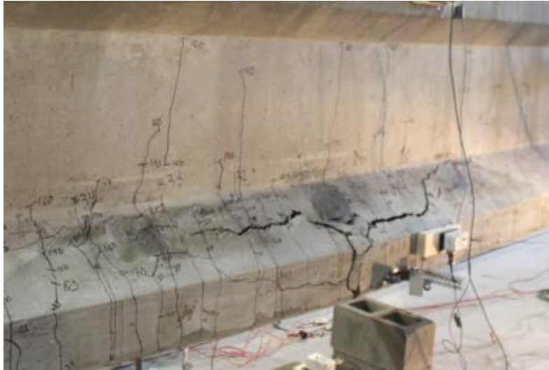
Figure 104- Flexural Cracks in Patch Concrete at Failure
