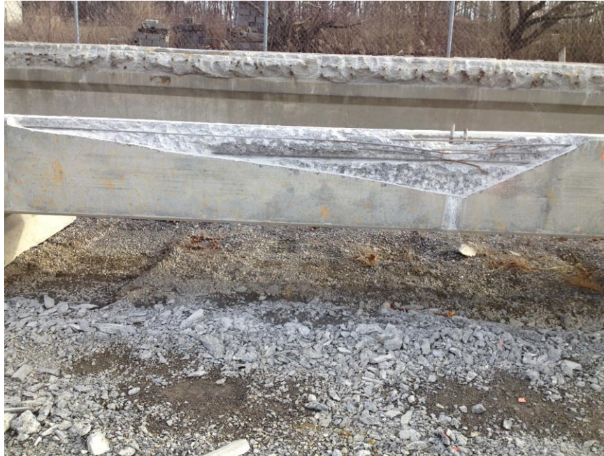
Figure 67- Girder D after Chipping and Saw Cutting
