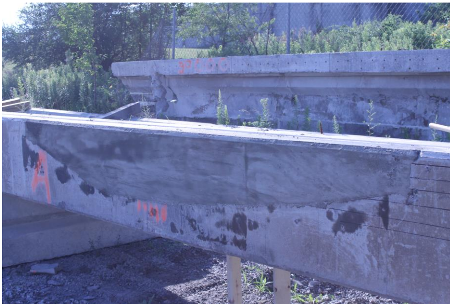
Figure 54- Completed Repair after Concrete Placement and Form Removal
