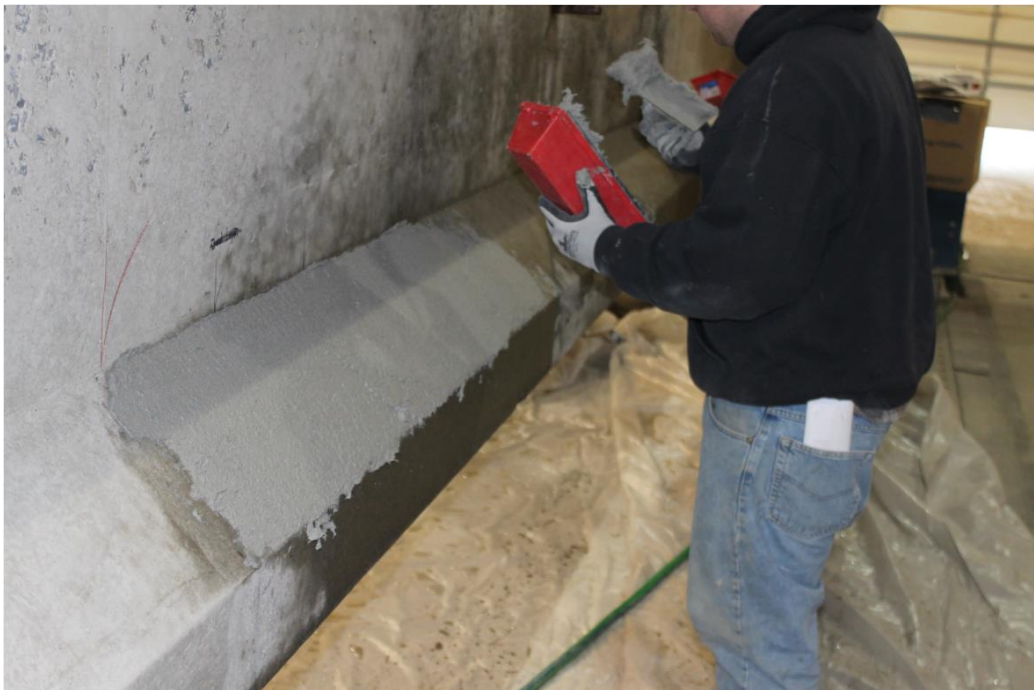
Figure 145- First Layer of FRCM Mortar
