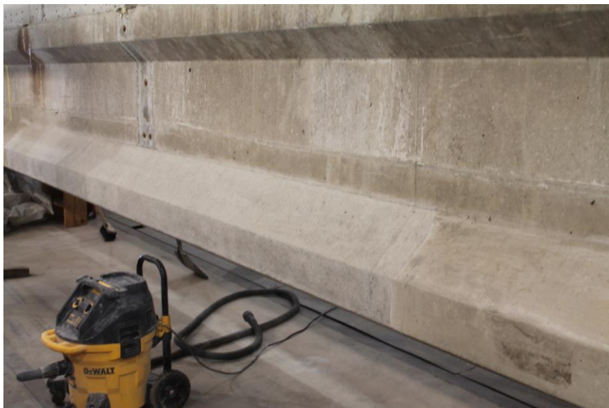
Figure 71- Repair Location after FRCM Surface Preparation
