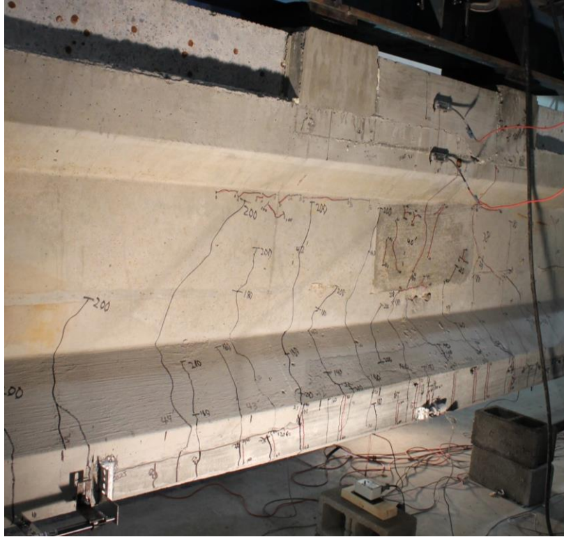
Figure 108- Test 4 Cracking Pattern at the Load Points during Iteration 1
