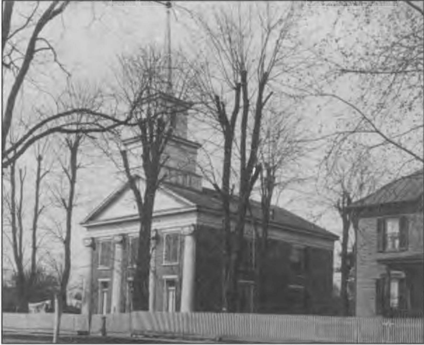
Figure 5. 1846 Methodist Church building.
