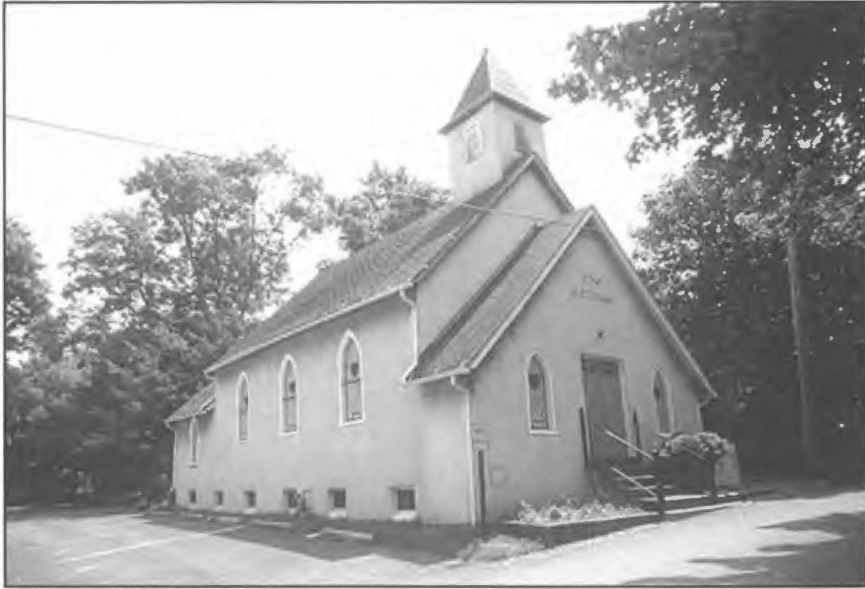
Figure 9. St. Paul AME Church still stands on the lot purchased in the 1870s. Though it is now covered with stucco, the original wood siding is apparently still contained within the structure.
