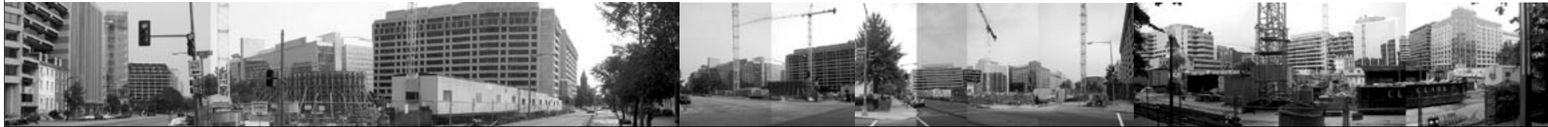
views of the site under construction September 2003
