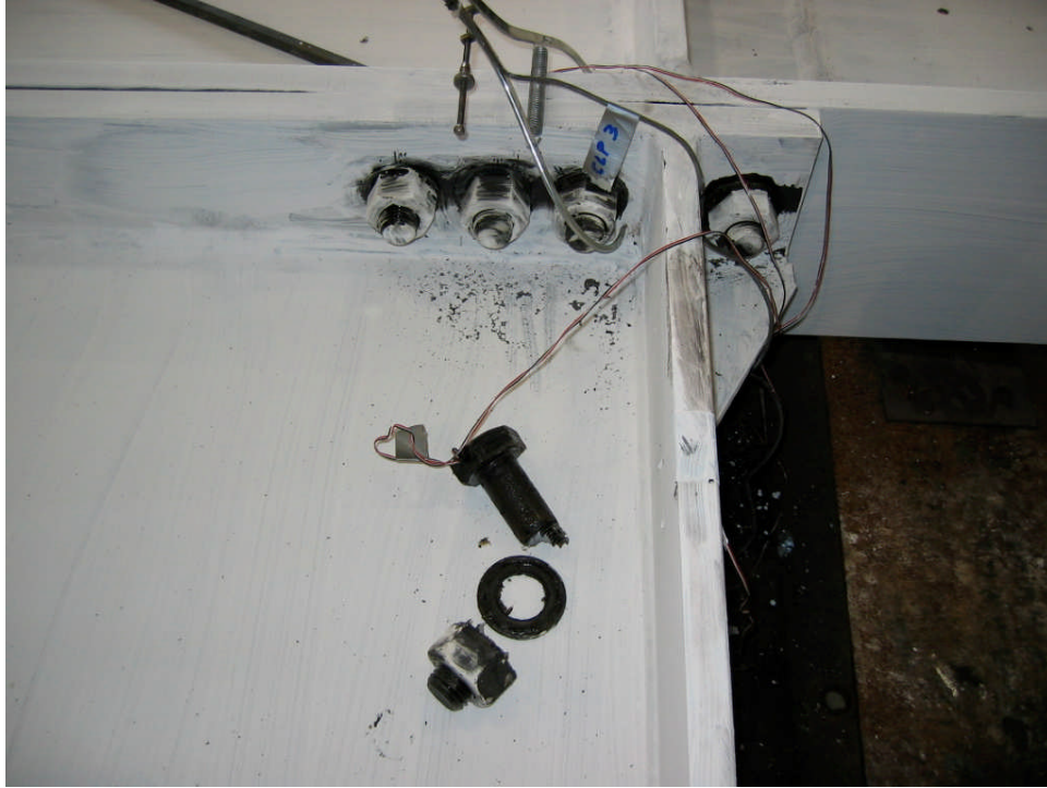
a) Bolt Rupture
