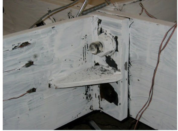
Far Flange at Bolt Rupture
