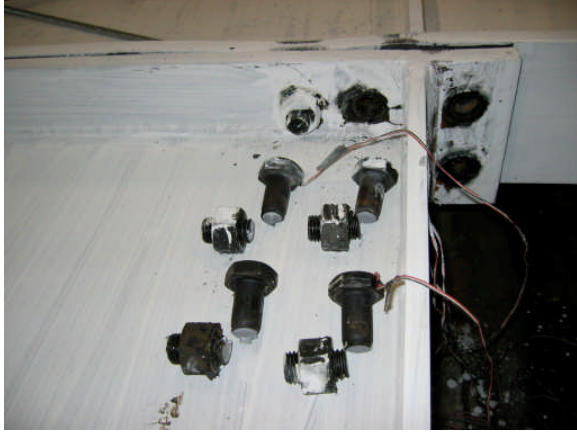
Bolt Rupture at Far Flange
