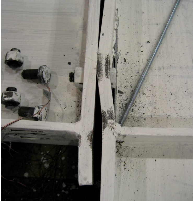
FIGURE 4.20: MRE1/2-1.0-10-60 A AFTER BOLT AND WELD RUPTURE
