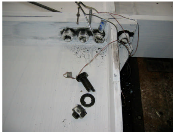
Far Flange with Ruptured Bolt
