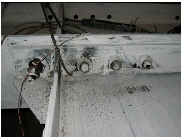
Near Flange At Ruptured Bolt
