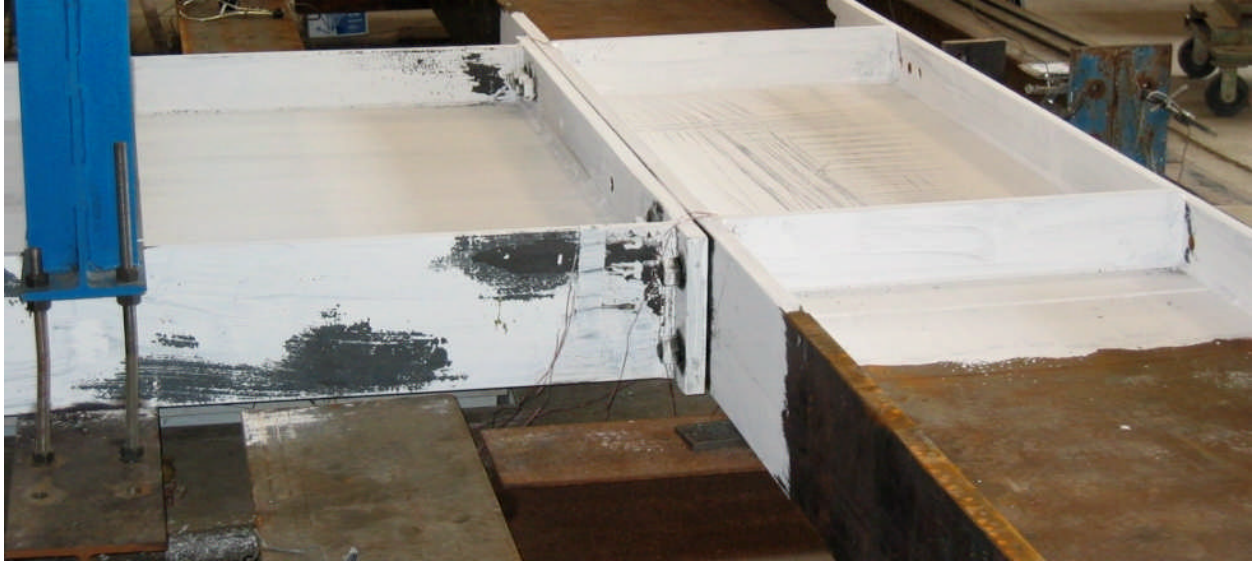
a) Overall View of Connection Region
