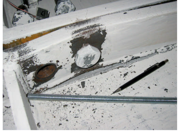
Weld Rupture at Far Flange
