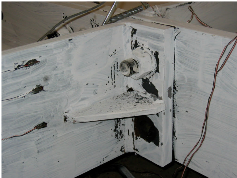
b) Area Near Ruptured Bolt
