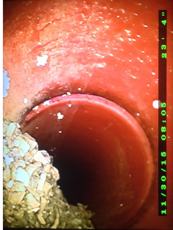
Figure 4: GCV System's Seventh Pipe
