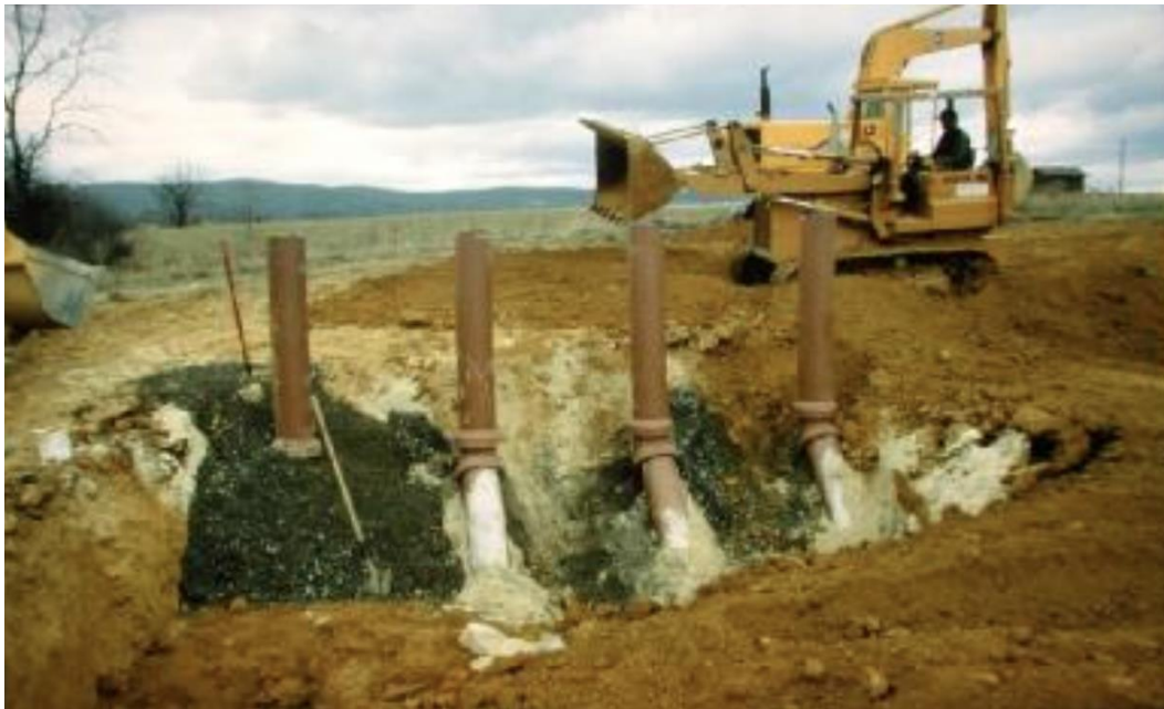
Figure 2-12: Vitrified Clay Pipes Used in the Solar CM House GCV System and the Gravel Backfill (photo by Robert Schubert)
