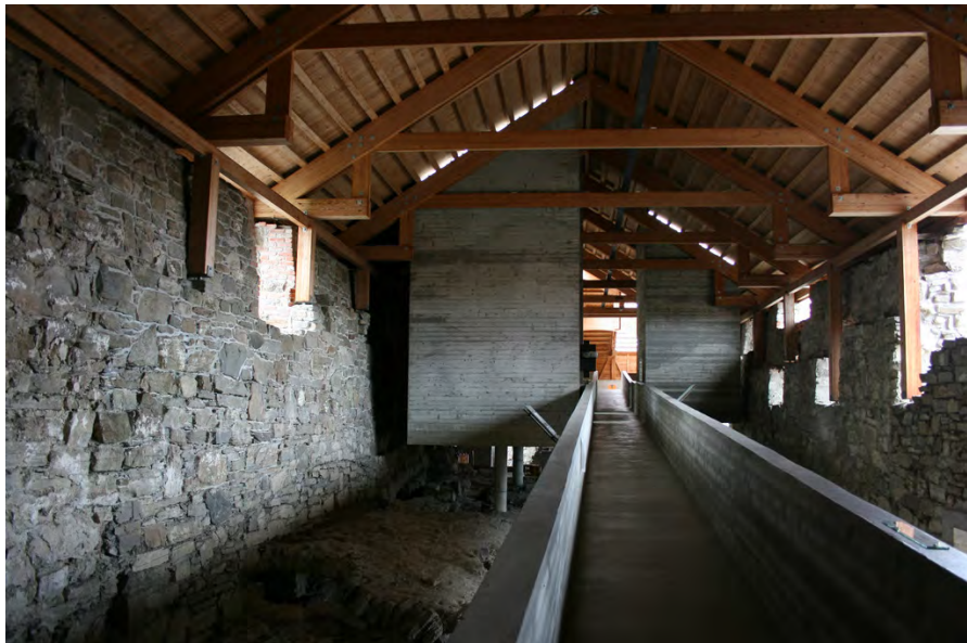
Slope going through the whole building
