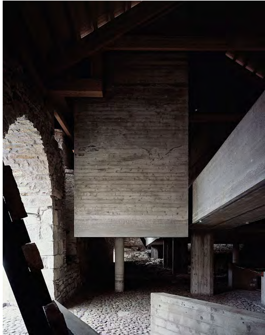
Gap between old structure and new design
