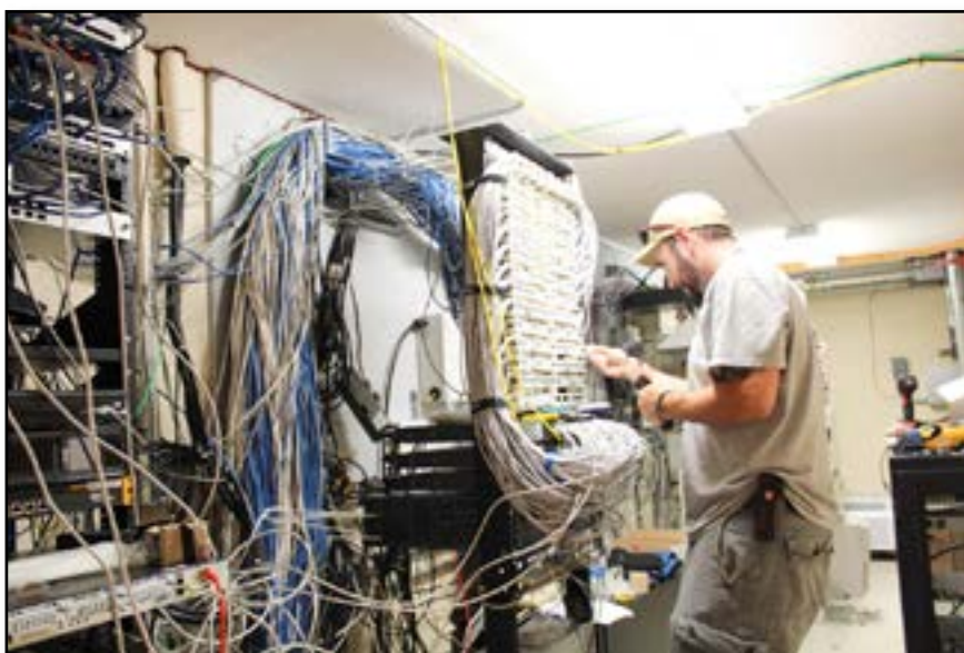
NI&S upgrades to technology infrastructure throughout campus improved connectivity and access to Virginia Tech's networks.
