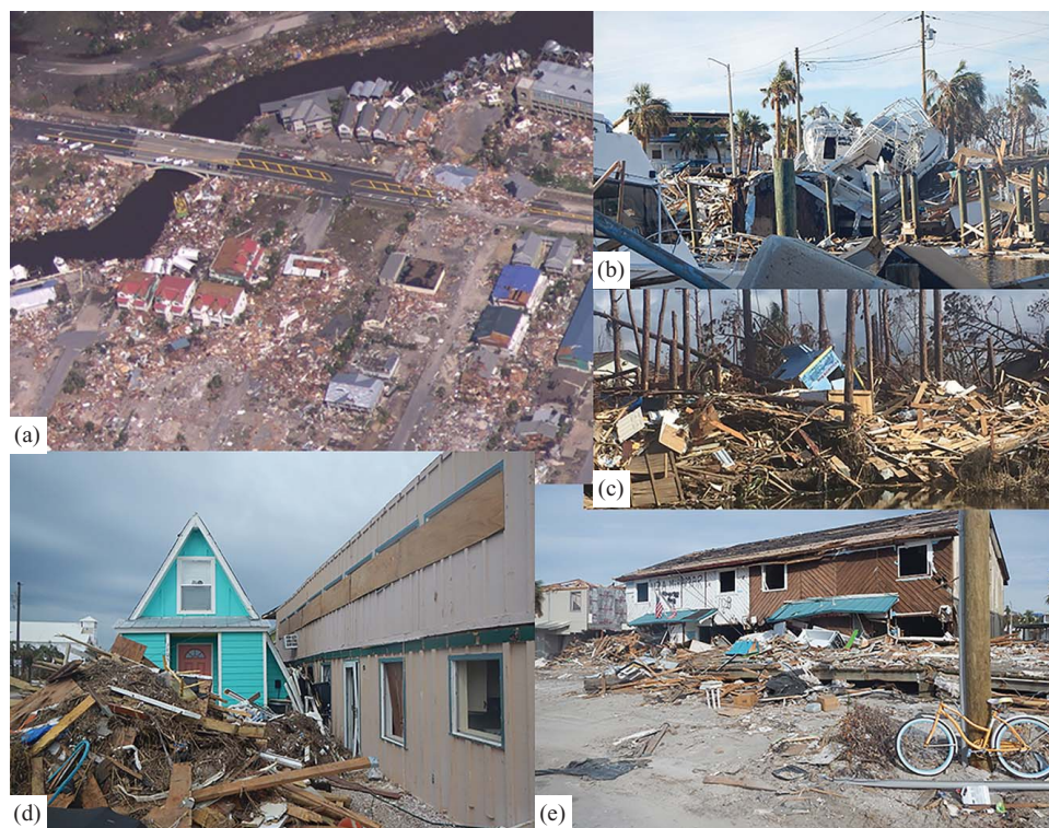
Fig. 14. (Color) Examples of debris transport and deposition: (a) Western Mexico Beach (image courtesy of NOAA), showing large debris piles; (b) boats and terrestrial debris; (c) waverunner rental shack and other debris in forested area; (d) large pile of woody debris and transported A-frame house grounded next to larger building; and (e) 34 m-long section of Mexico Beach Pier deck grounded against houses. (Images (b–e) by authors.)
