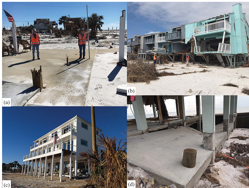
Fig. 8. (Color) Examples of structural damage: (a) complete failure of pile elevated house (DS6); (b) severe damage to beachfront pile elevated row houses (DS5); (c) minor damage to Sand Palace (DS3); and (d) scour and partial failure of concrete floor pad underneath pile elevated house (DS5). (Images by authors.)
