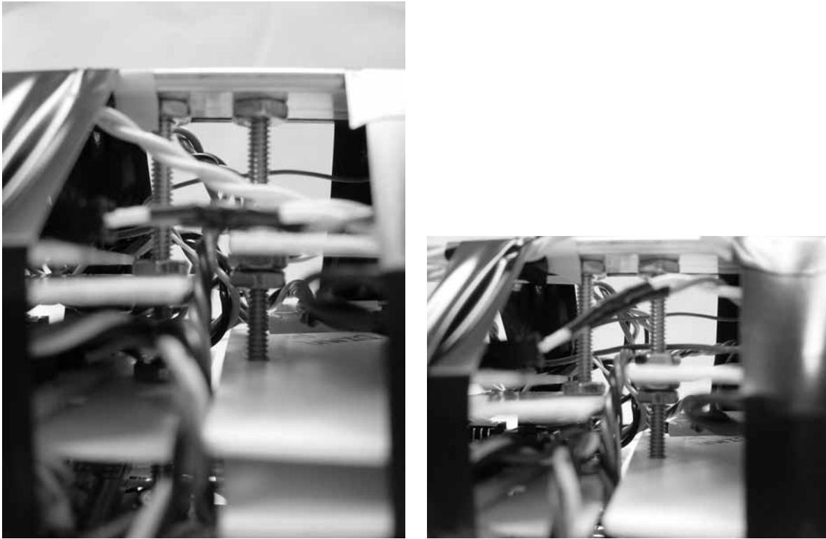
Figure 2.13: Card mounting, close-up view displays styrene cards and nuts securing them along support screws
