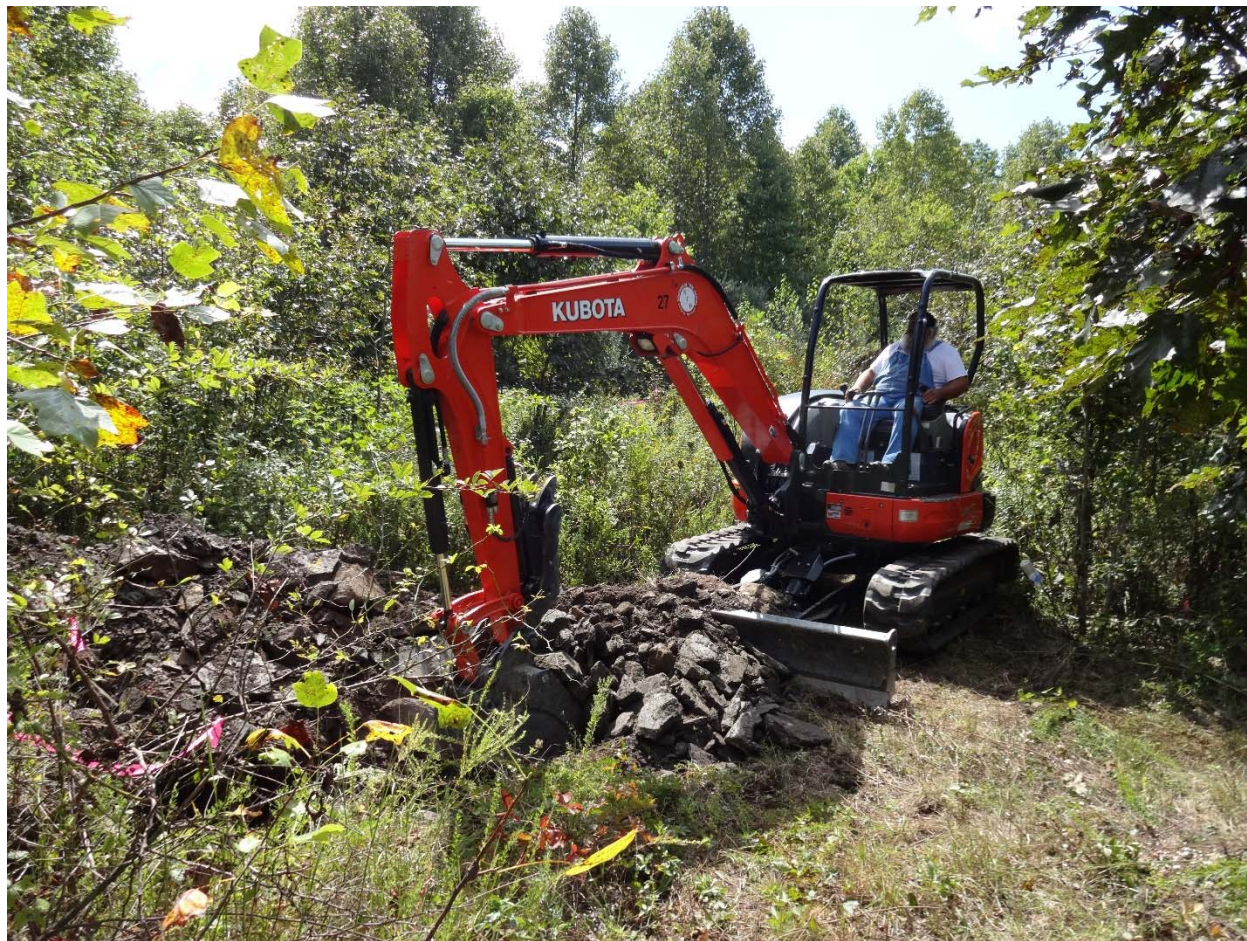
Figure 1. Soil observation and sampling pit being excavated by Dan Early in a pure siltstone (SiS) plot in the Rock Mix Experiment in September 2016. Excavator traffic was limited to the alleyways between plots and the soil pit face was aligned to allow for optimal photography.
