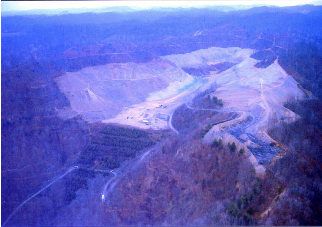
Figure 2. The mine site viewed from southeast in early 2002 (from Showalter 2005).
