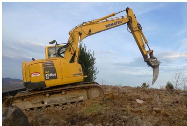
Photo 5. An excavator outfitted with a ripping tooth can loosen compacted soils on slopes that are too steep for a dozer.
