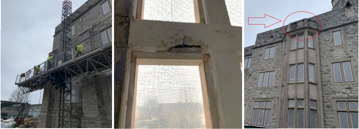
Figure 6.1: Left images shows workers at height inspecting and repairing building envelope. The center image shows damages on the precast concrete envelope due to lack of periodic inspection. The right image shows building exterior envelope requiring inspection and repair at height during construction and major renovation.
