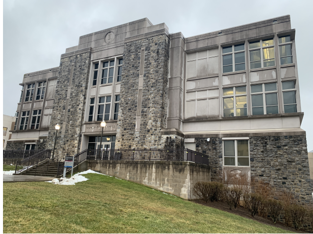
Figure 6.3: Image of Bishop-Favrao Hall which is utilized as a test case for this work.
