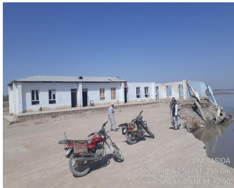
Figure 2. A school constructed in an Amu Darya river flood plain in Afghanistan and partially destroyed by flooding. This image was provided by Development Monitors LLC.
