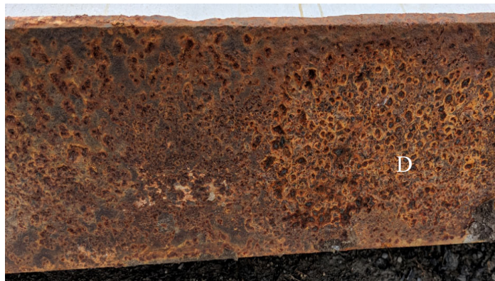
II. Severe Grade of Rust
