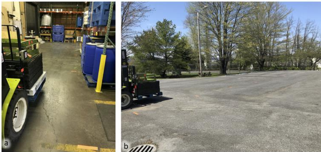
Figure 18. Investigated road conditions: a) concrete, b) asphalt
