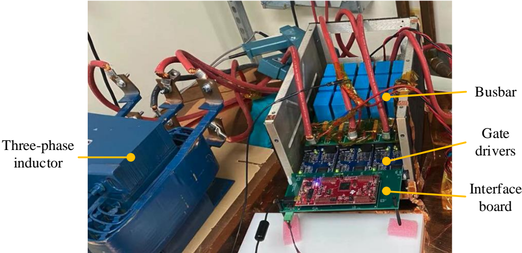
Fig. 4- 27. Test setup for three-phase continuous testing.
