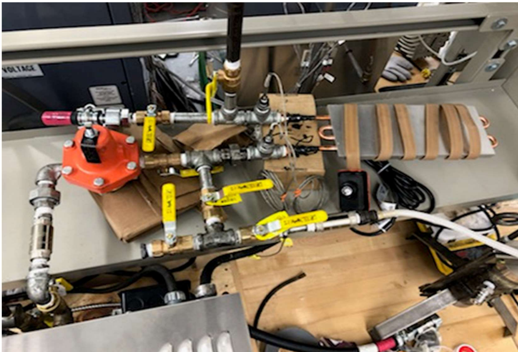
Figure 9: Piping components prior to being insulated. Piping is shown leaving the boiler and passing through the pressure regulating valve, shutoff valves, heat sink plate, and finally the flexible hose.
