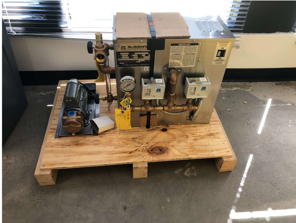
Figure 7: The electric steam boiler purchased for use in the drying experiments.
