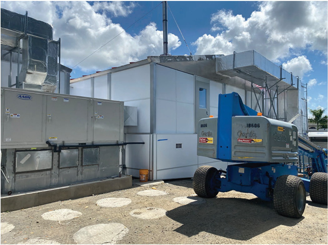
Figure 12.3 Modular Hospital on St. Croix Under Construction
