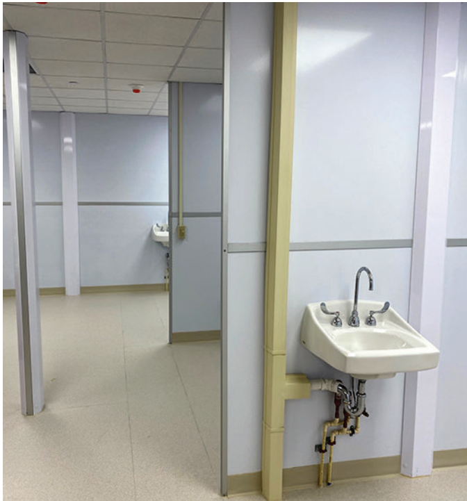
Figure 12.2 Emergency Room in a Modular Hospital on St. Thomas
