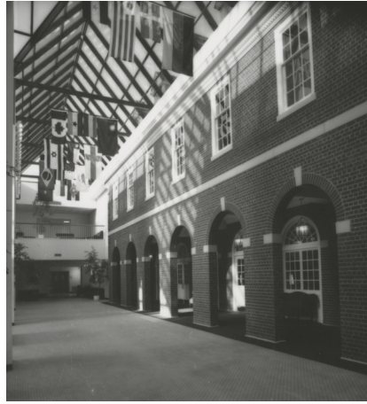
The 1990s renovation to Squires Student Center reveals the original 1930s façade
