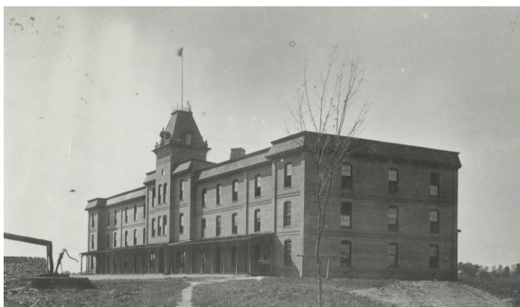
Barracks No. 1, later Lane Hall
