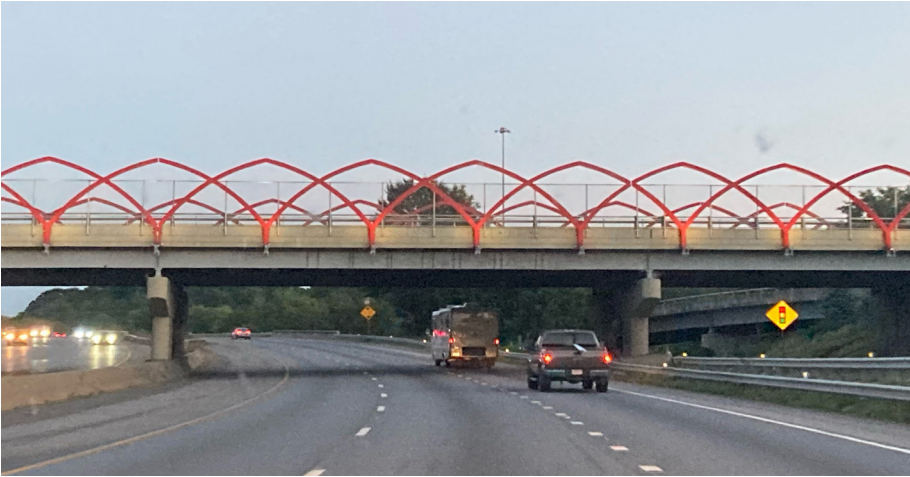
Figure 9.6. "Washington Street Bridge Gateway"
