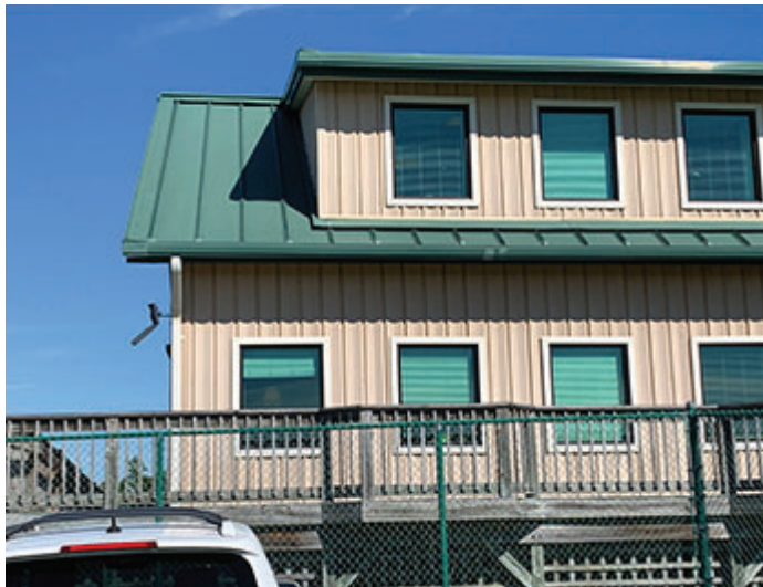
METAL SIDING & ROOFING
